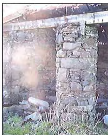
Radiused masonry elements
