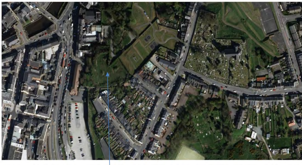
Fig. 5. Aerial view of the site, taking in the surrounding context, which is characterised, almost exclusively, by terraced buildings with no in-curtilage parking provision and almost all parking provided on-street.
