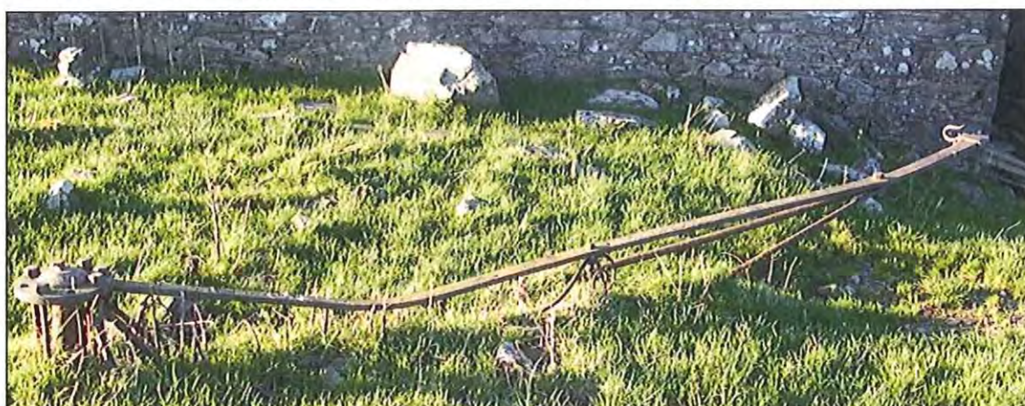
Horse walk track, halter, hub and gearing, rear wall of Mill
