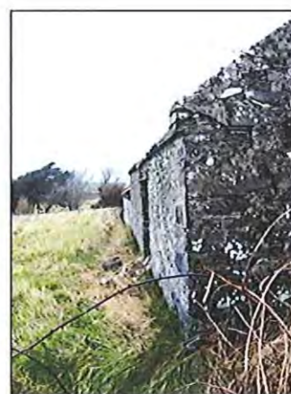
Front wall, eaves and gable 'knee'
