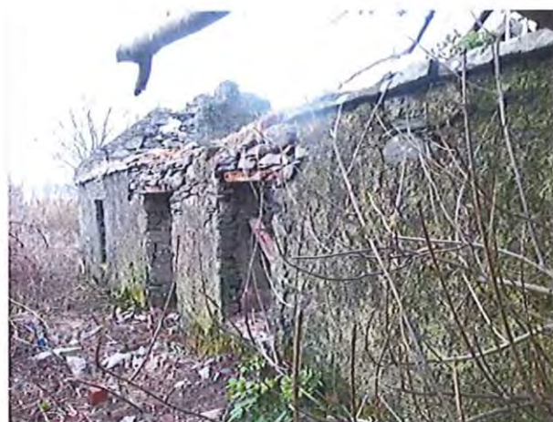
Rear wall intact to eaves level
