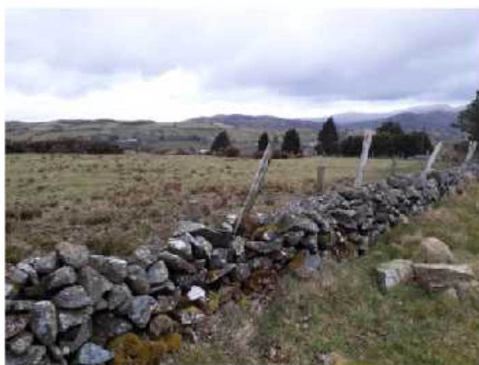
View along the eastern boundary
