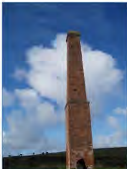
Red brick Chimney
