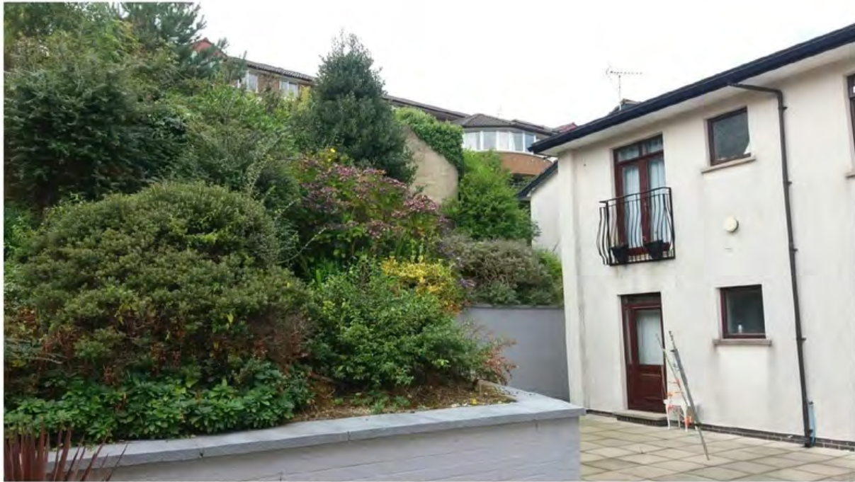
3) View of existing balcony on rear elevation
