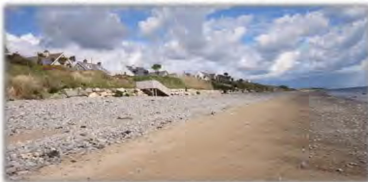
Photo 2 – Existing hard defences in the vicinity of Windmill Road
