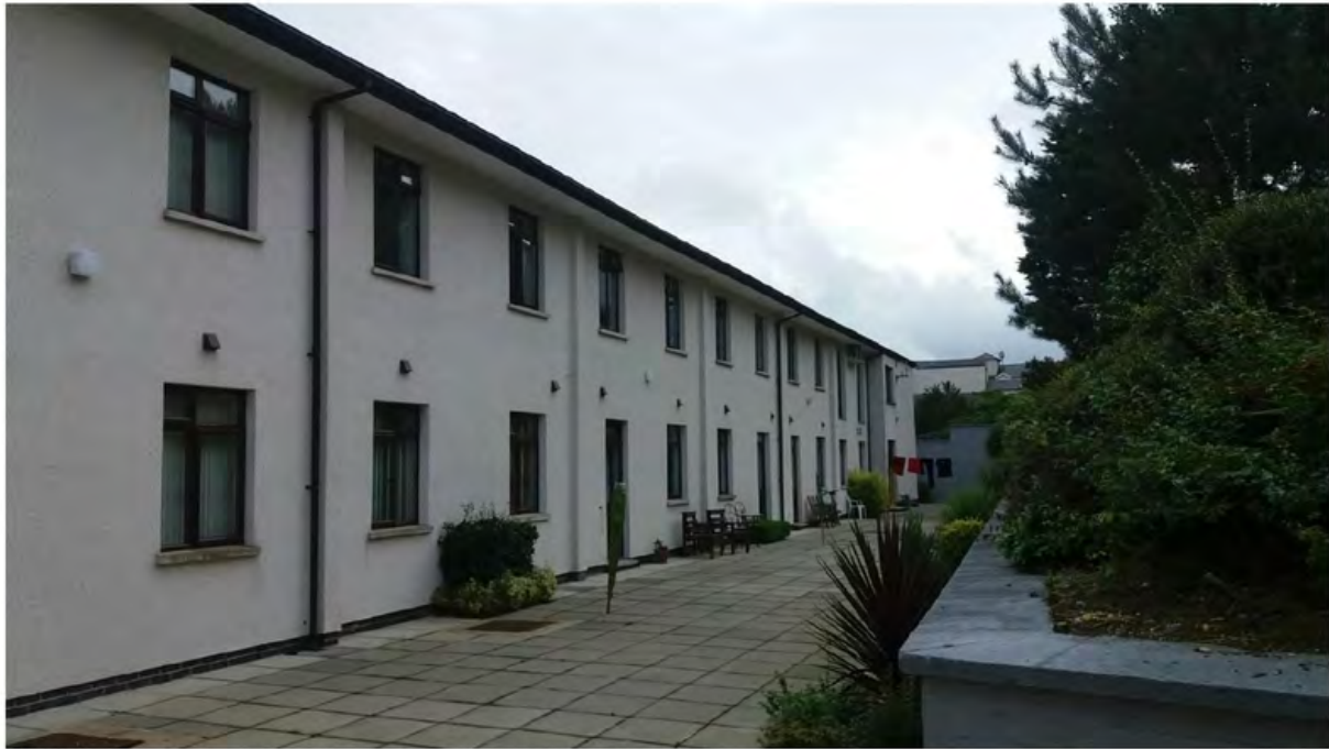
4) View looking South East from rear elevation
