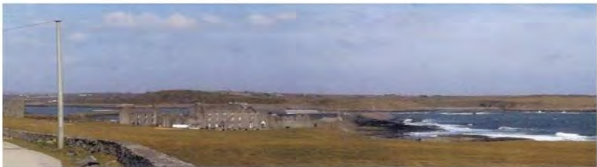
Existing View from Castle Place Ardglass
