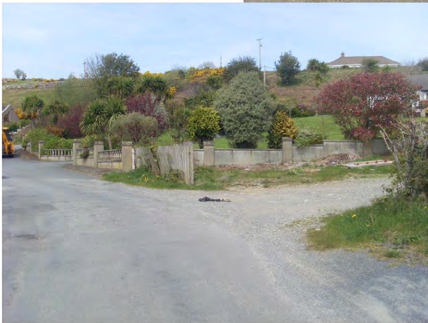
Site entrance and the boundary wall of No. 31
