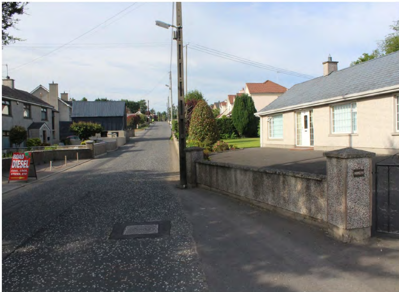
Fig. 4 – Image showing the lack of sight line to the north of the existing farm entrance. The existing access is clearly not suitable for increased use.
