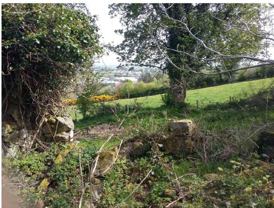
Image 3 Walls tumbled to the East
