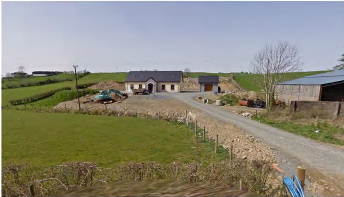
Figure 13 Single storey roadside development with visually dominant driveway
