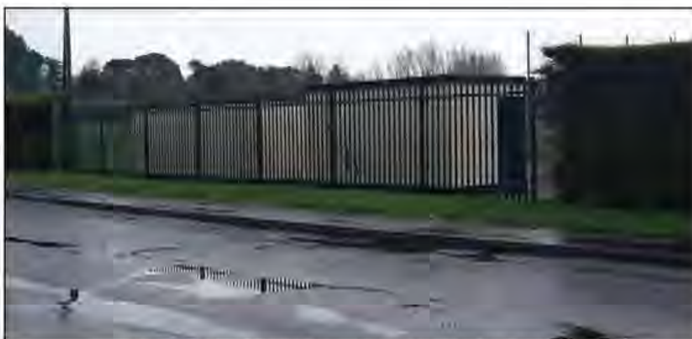
Figure 1 - Existing View of Palisade Fence and Mobile Containers
