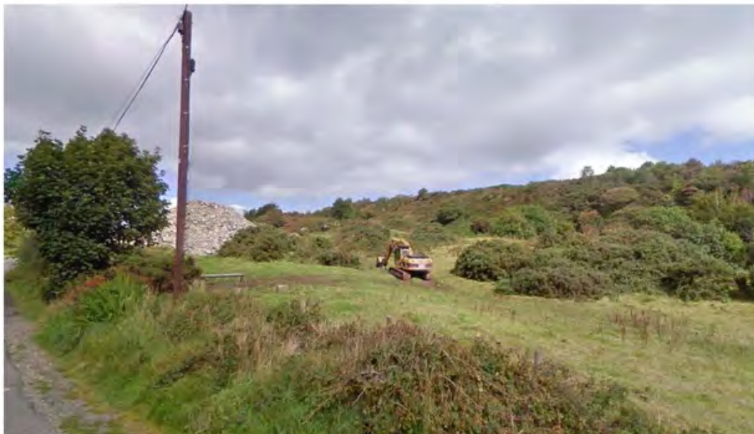
Figure 6 View of proposed site.
