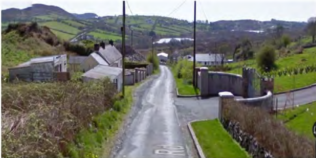
Figure 4 Existing roadside residential property north of the application site.
