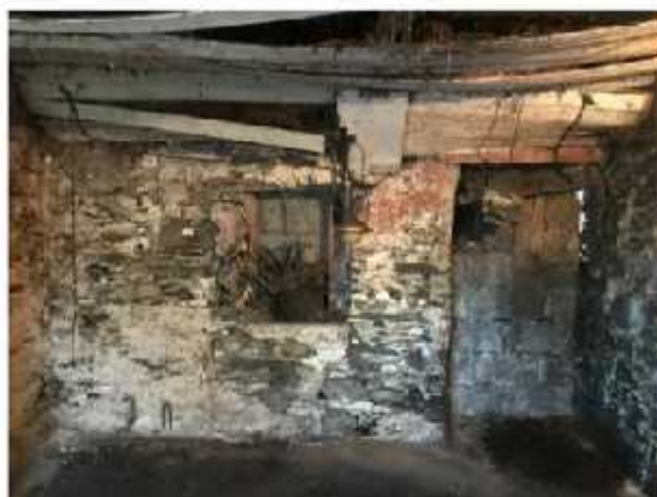
Photos 3 & 4 – Internal view of external southern wall with blocked up door and window opening to larger room. External structural wall are substantially intact.
