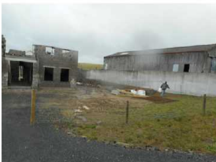
Photo 12 – Byre and new dwelling under construction
