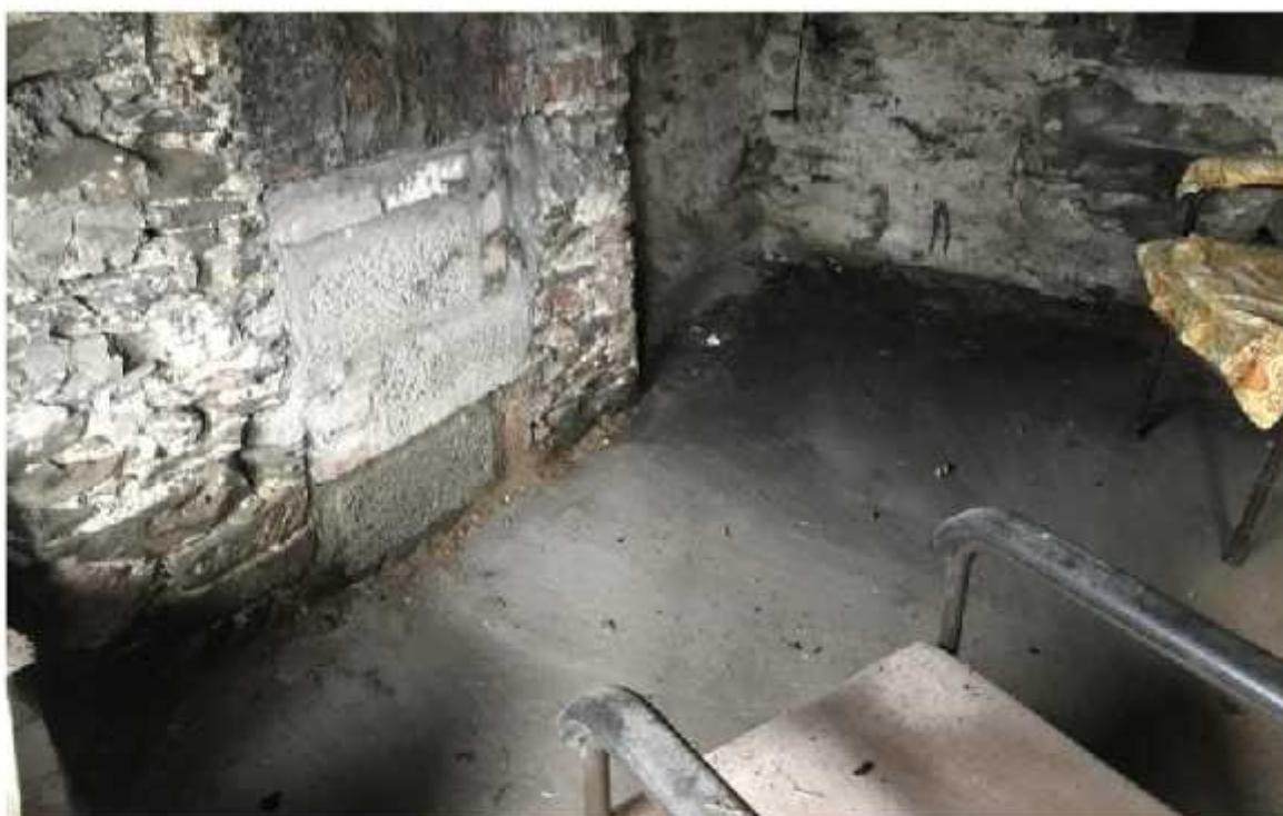
Photo 21 – Concrete floor to main room
