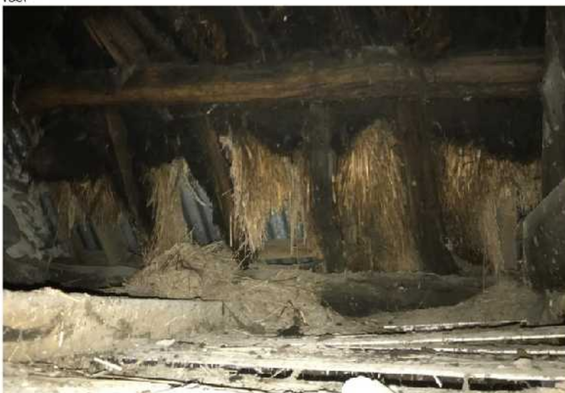
Photo 9 – Detail of thatched roof above ceiling
