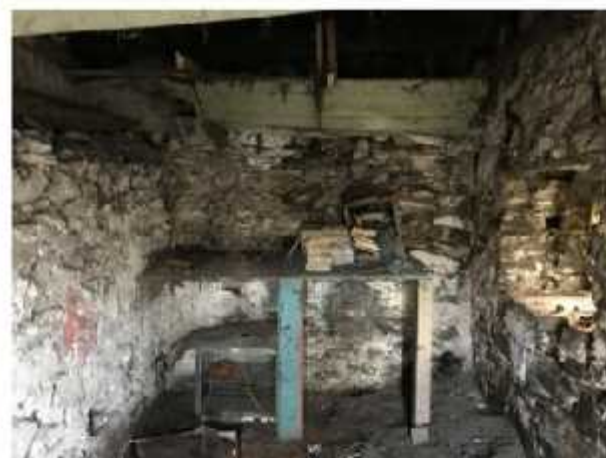
Photos 3 & 4 – Internal view of external southern wall with blocked up door and window opening to larger room. External structural wall are substantially intact.
