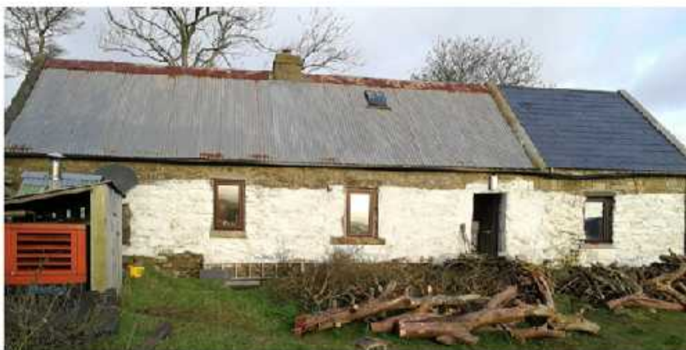
Photo showing front elevation.
