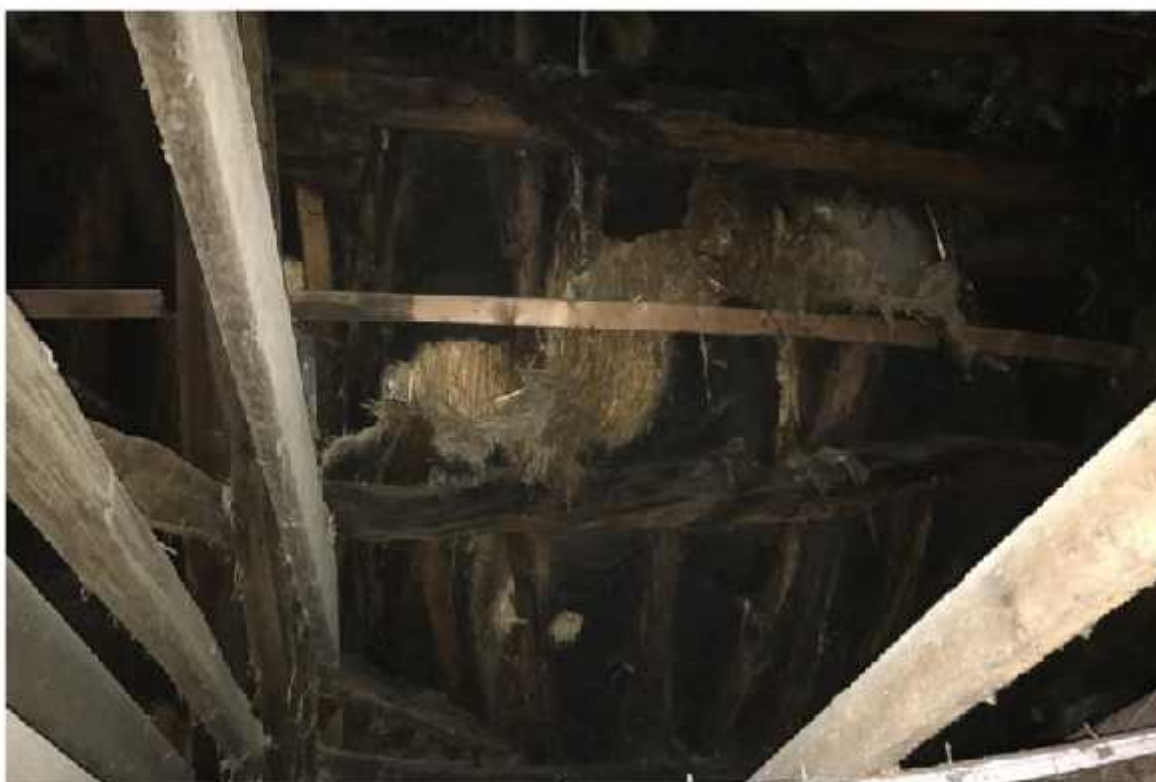
Photo 8 – Thatched roof below the metal roof
