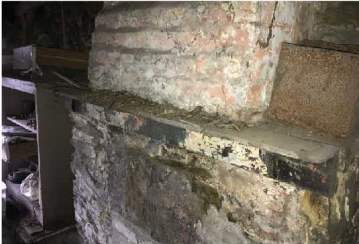
Photo 12 – Wooden mantelpiece over blocked up fireplace & hearth
