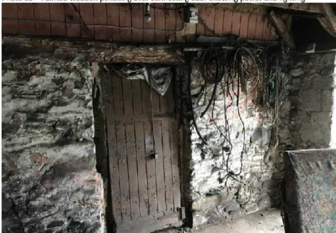
Photo 11 – Connecting wooden door between each room
