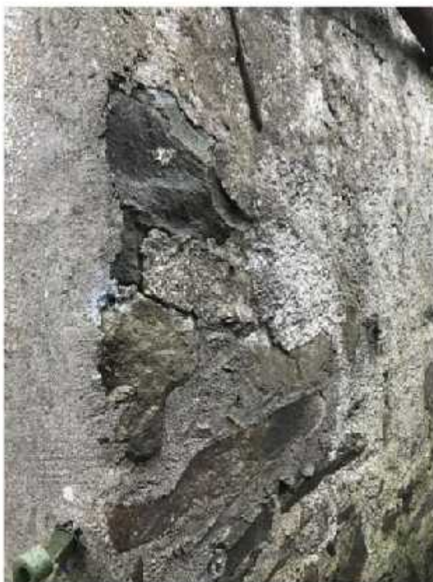
Photo 4 – Detail of external wall showing lime render on rubble stone
