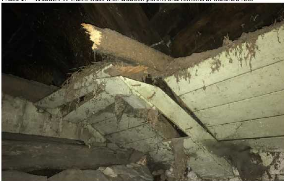
Photo 18 – Painted wooden ceiling panelling and wooden trusses
