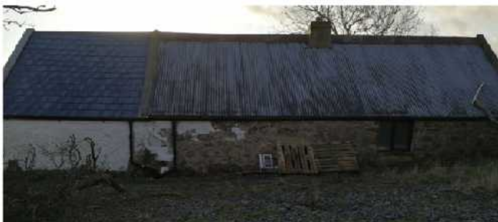
Photo showing rear elevation.
