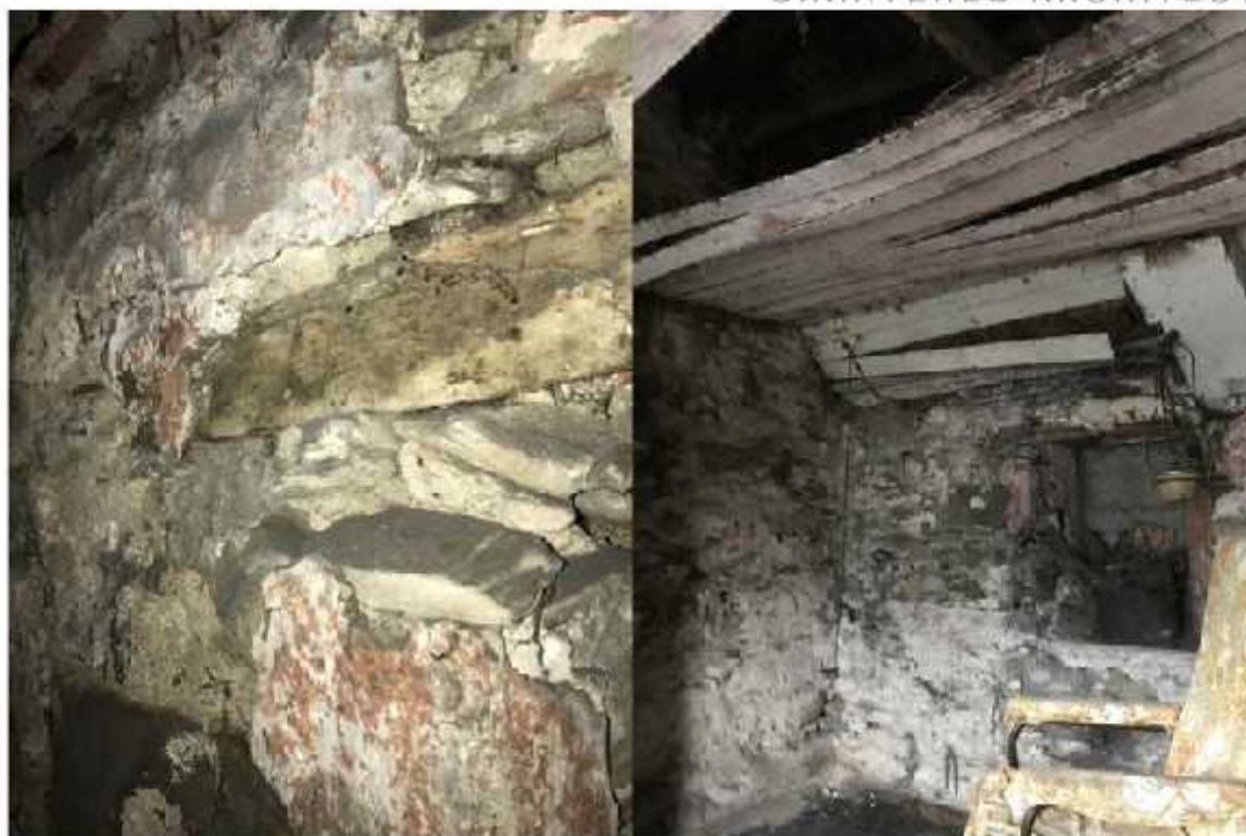
Photos 14 & 15 – Internal plaster over stonewalls, painted wooded boarded ceiling
