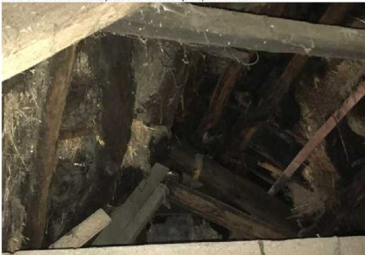
Photo 13 – Wooden truss roof with remains of thatched roof
