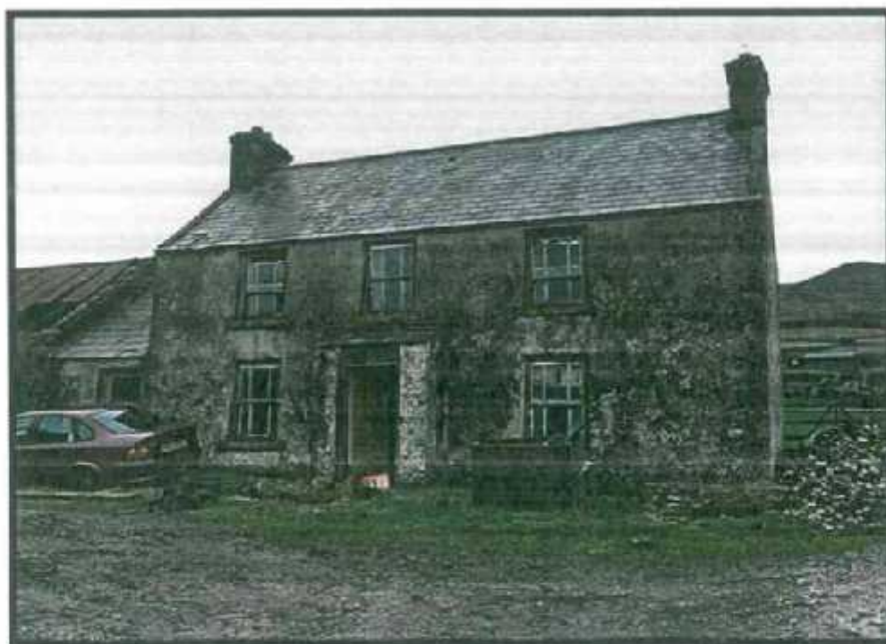
The existing dwelling at No.173 Head Road
