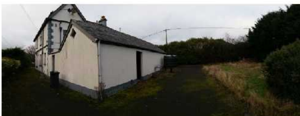
Rear and S Elevation of No. 58
