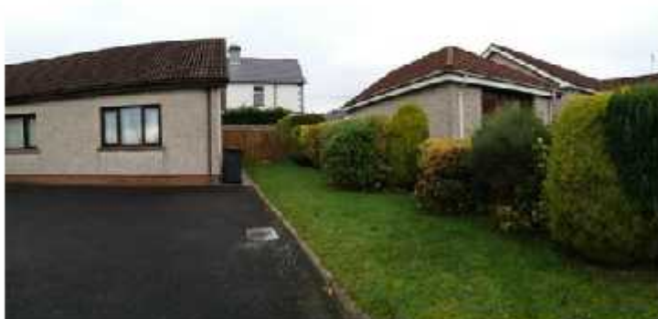
Existing building to rear of 2 and 4 Glenpatrick Lawns
