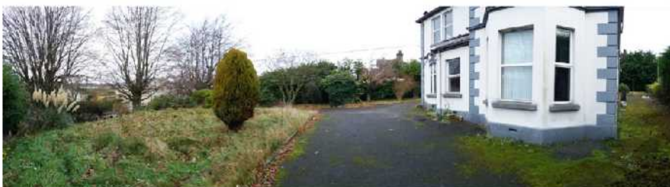
Front elevation and front garden of No. 58 Armagh Road
