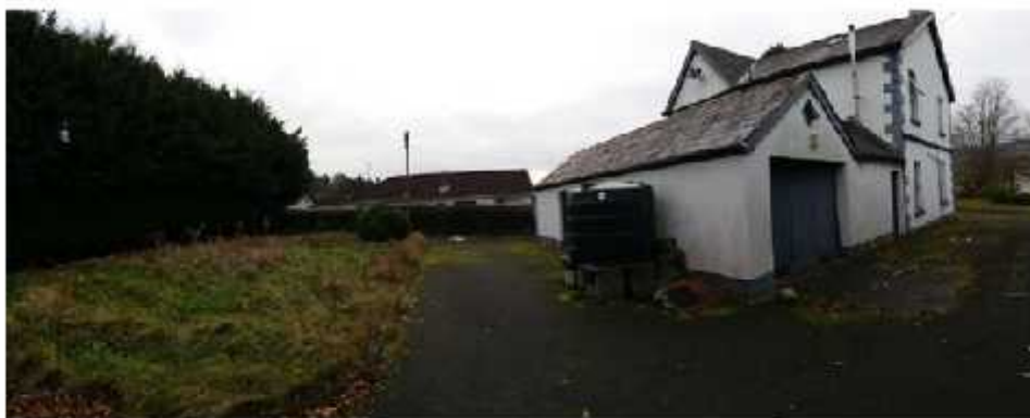
Rear and N Elevation of No. 58
