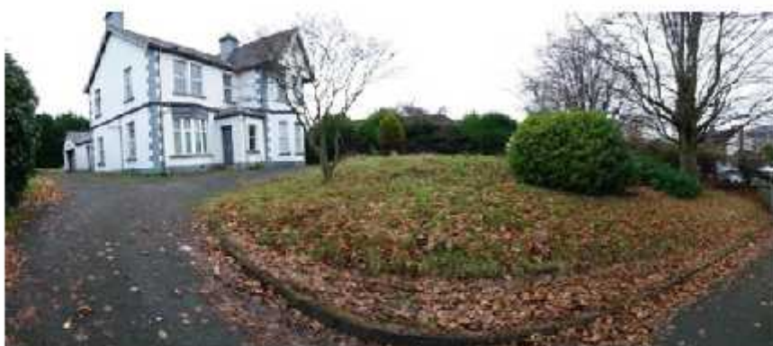
Existing dwelling at No. 58
