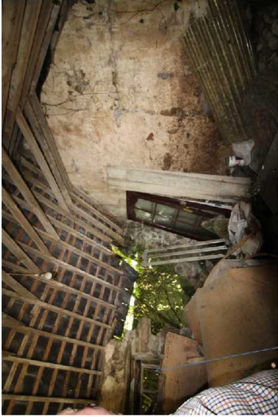
Window opening with frame intact. This frame is consistent with residential use of the building.
