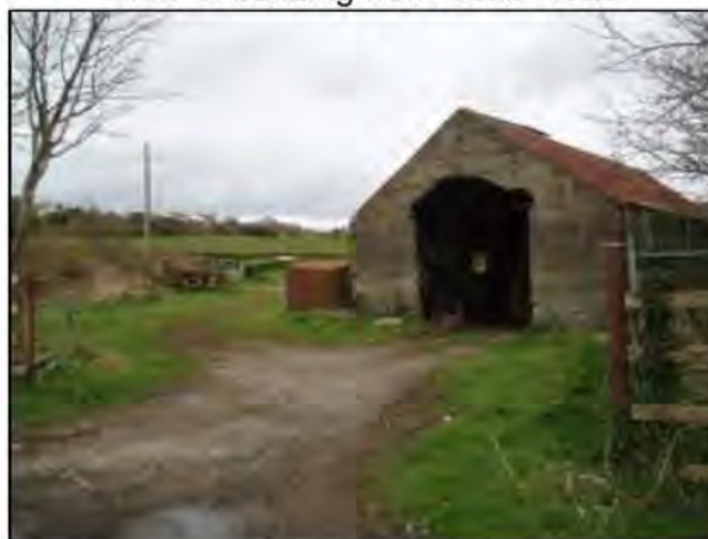
View of building from Scrib Road
