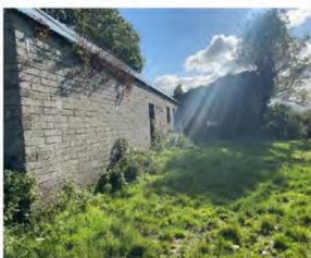
Evidence of breeze block rebuild
