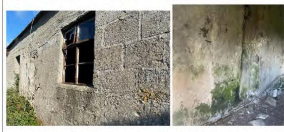
The only window, does not look original and surrounded by concrete block which would have been added at a later date.
