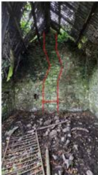
outline of previous chimney flue in red
