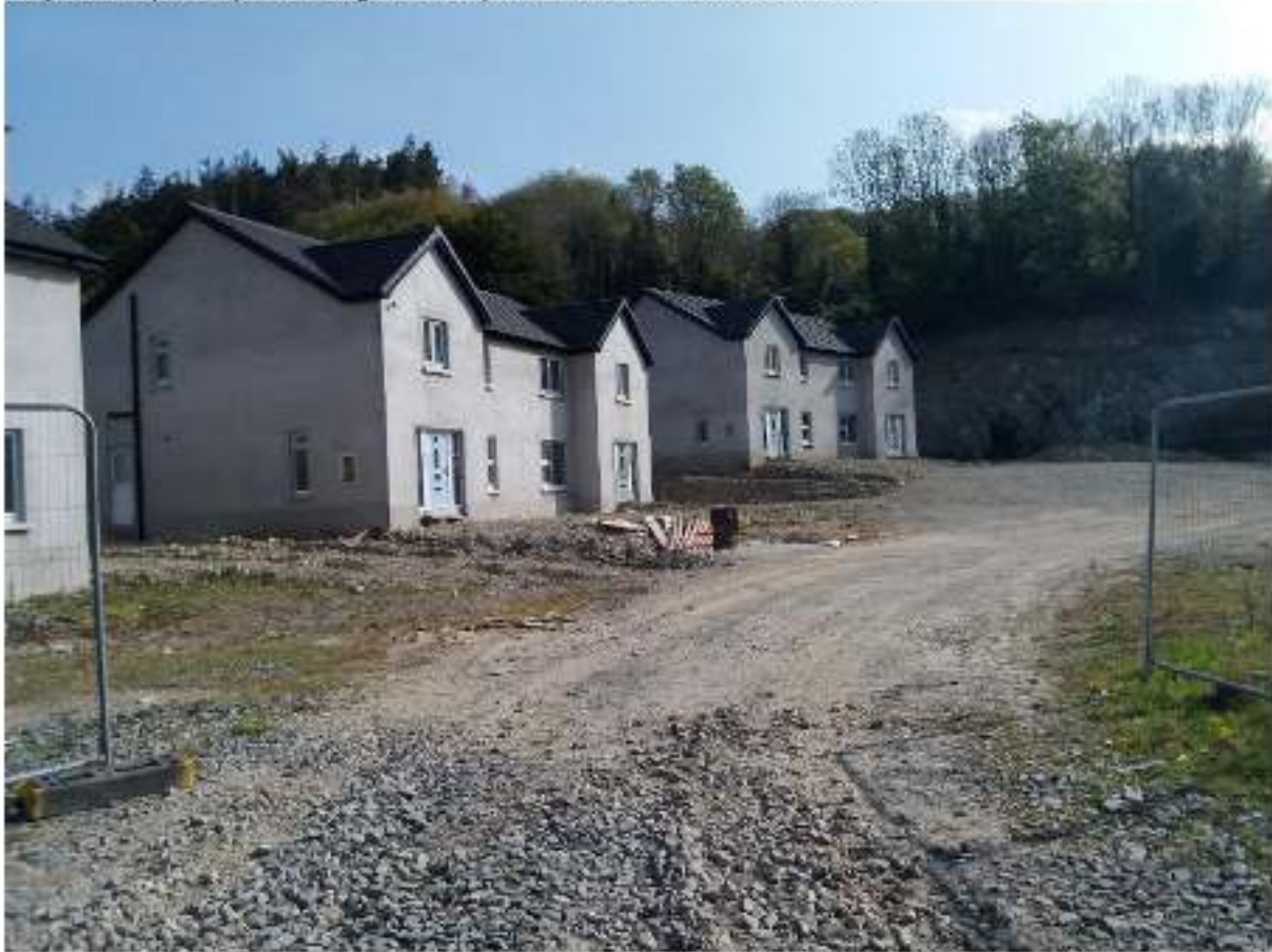
Adjacent (north) housing development under construction:
