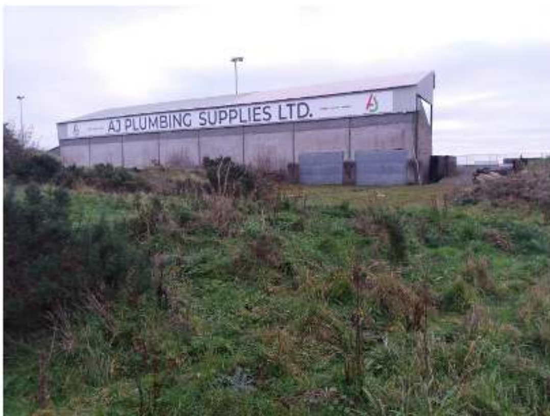
View from the application site towards existing terrace structure
