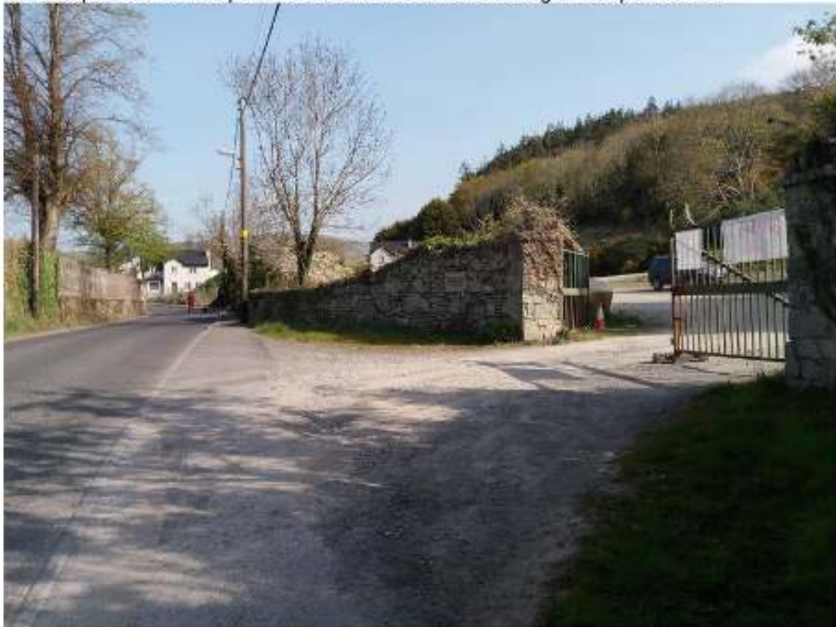
Access point off Greenpark Road and views north along Greenpark Road:
