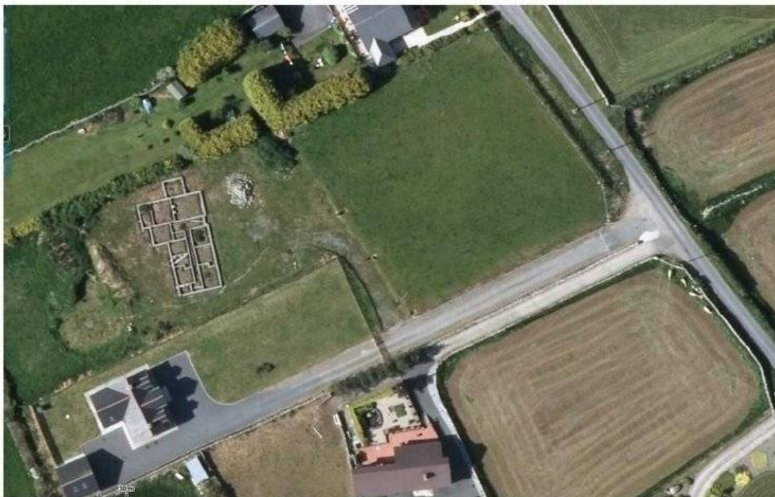
It is clear from the site inspection, aerial images and Google streetview images that the access works are still not in place in 2016.
