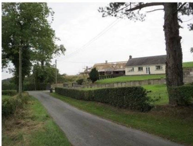
View of No. 37 and its replacement under construction
