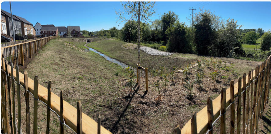
Example of SuDS at Belmont Hall, Antrim. (courtesy of Antrim Construction Company)
