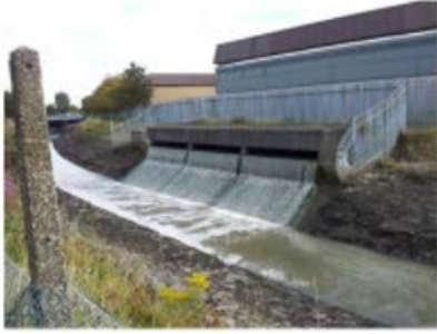
Unsatisfactory Intermittent Discharges (UIDs)
