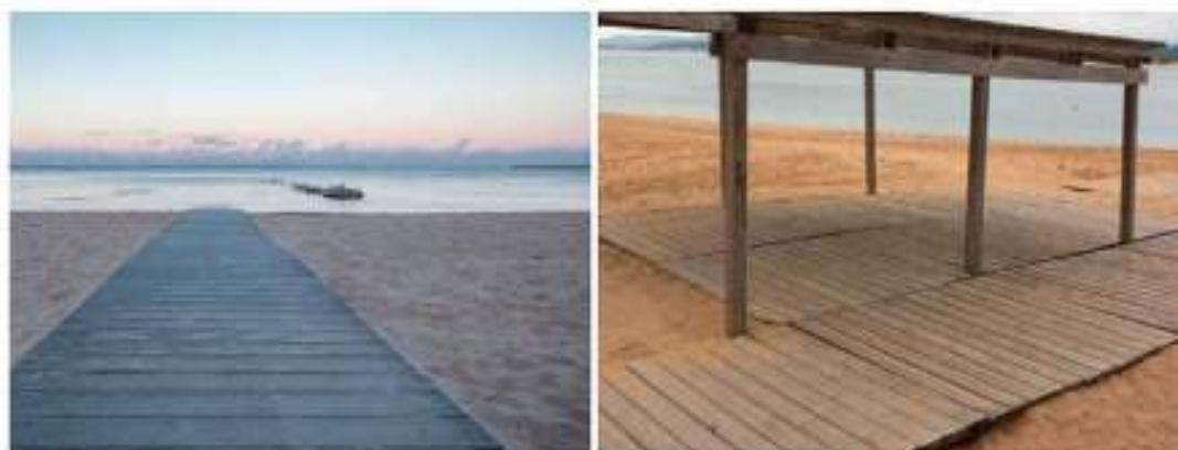
Figure 5: (L) Modified Wood Accessible Boardwalk; (R) Accessible Boardwalk and Shelter
