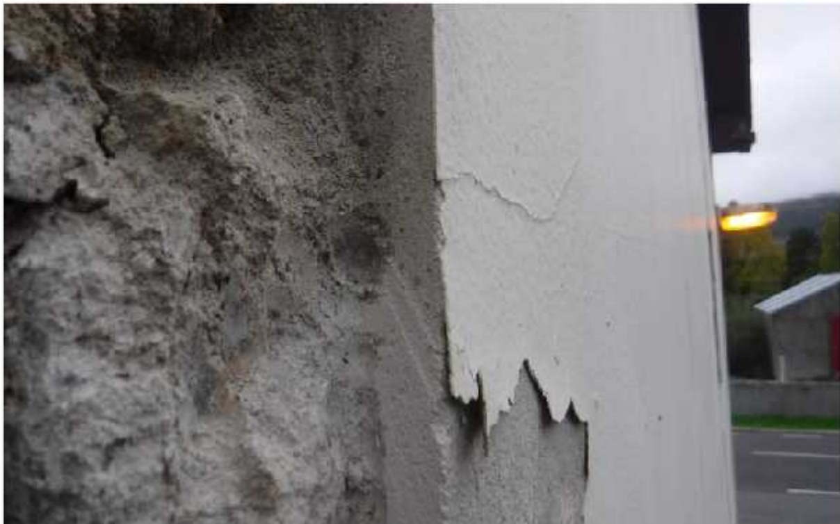
Figure 6 - Close up of Crack at Breakout 1 Showing Minimal Depth of Cracking
