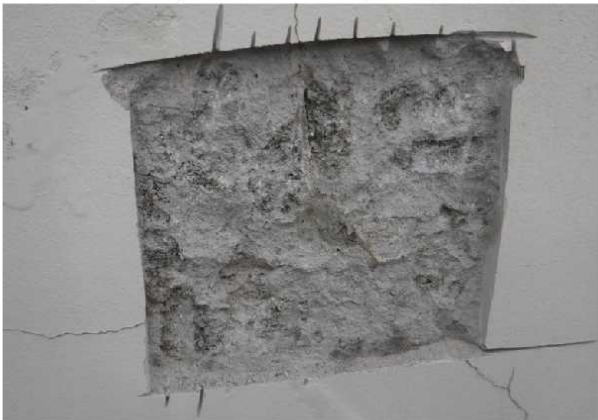
Figure 6 - Close up of Crack at Breakout 1 Showing Minimal Depth of Cracking
