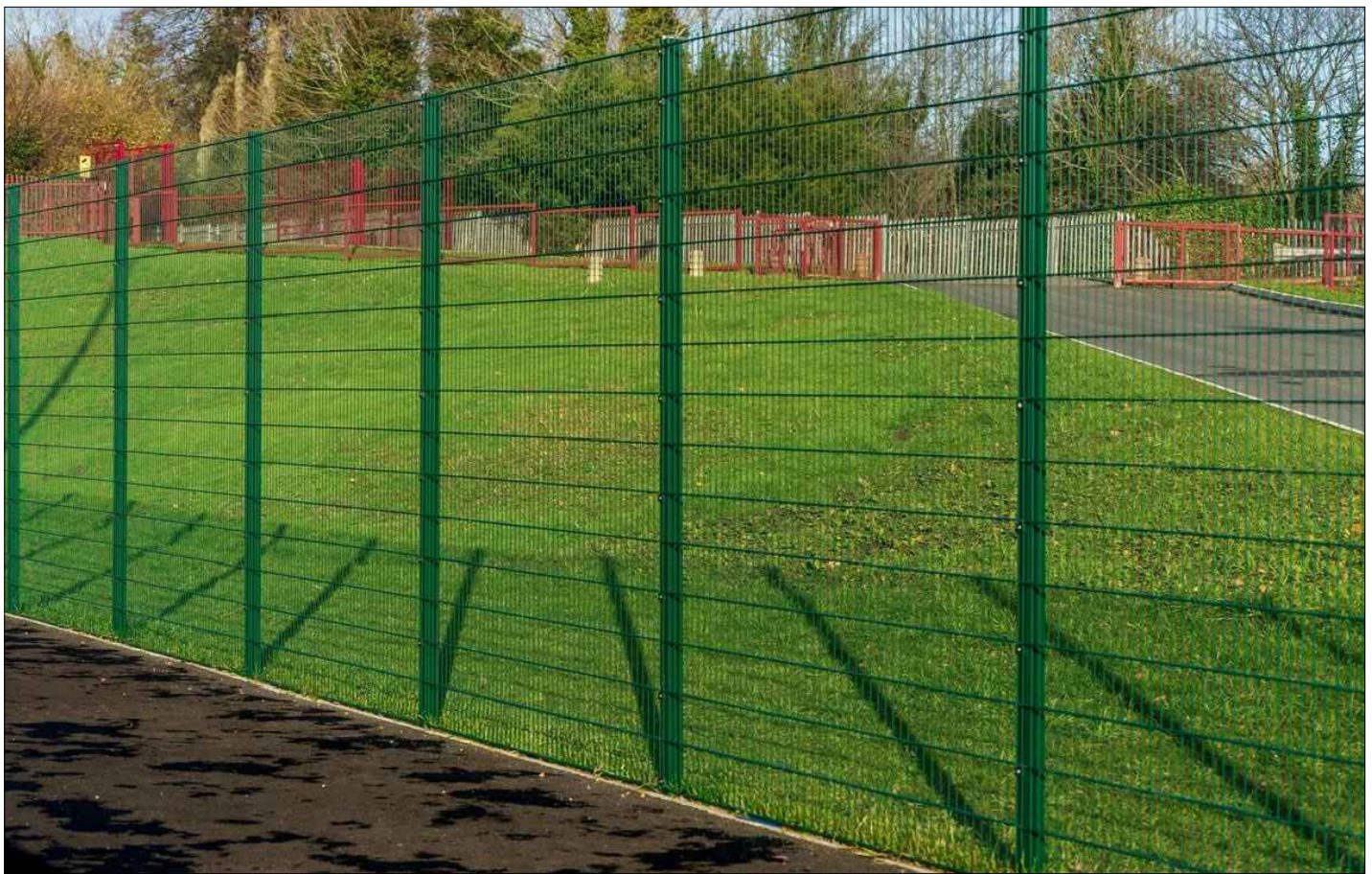
2.4m Perimeter Fencing / Gates
