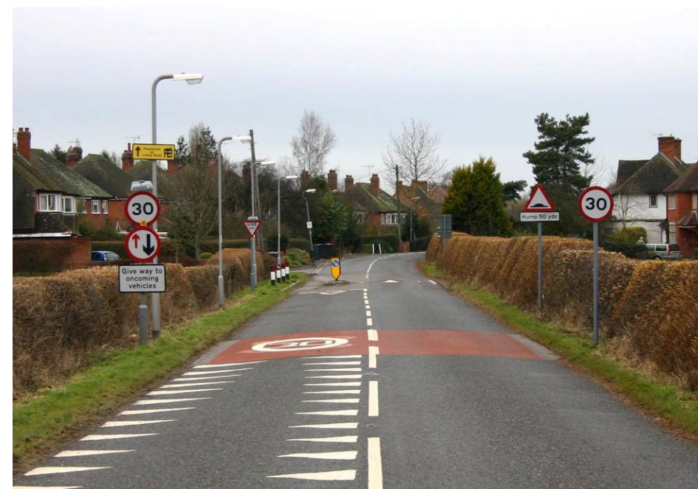
Road markings, signage and speed humps
