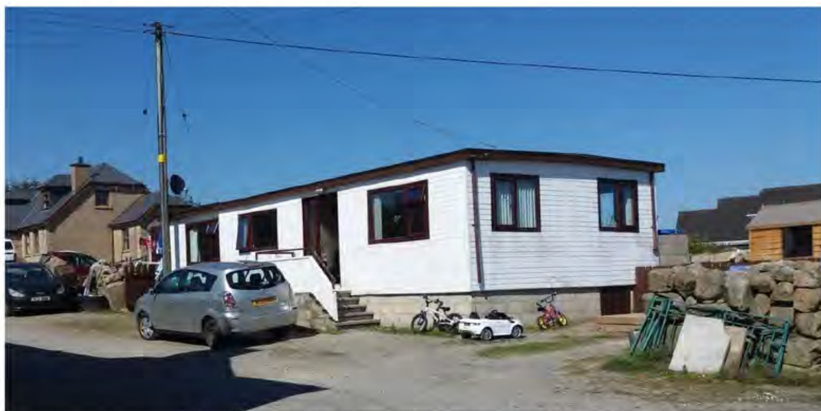
Existing building of temporary construction (No. 61B)
