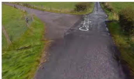
Photo 8 Paved access with adequate width to facilitate vehicle movements. Adequate visibility to the SW and NE
