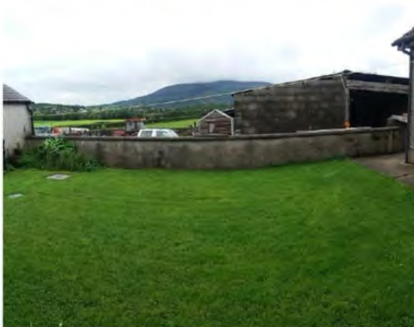
Existing buildings at No.73 Newtown Rd
