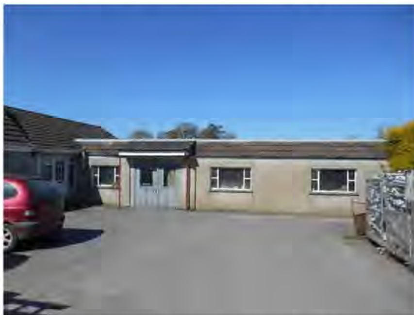
Photograph 1: 103a Manse Road. Window Frame workshop viewed from the south.
