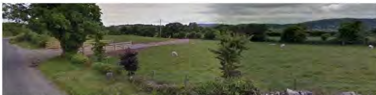
P/2014/0217/F; an application site located immediately adjacent to the roadside, with minimal screening in existence. The agricultural building will be clearly visible along a not insignificant stretch of Chapel Road, Ballyholland.
