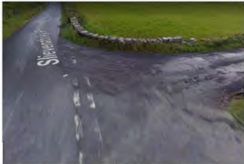
Photo 1 Carnigagh Road Slievenabley Road priority junction
