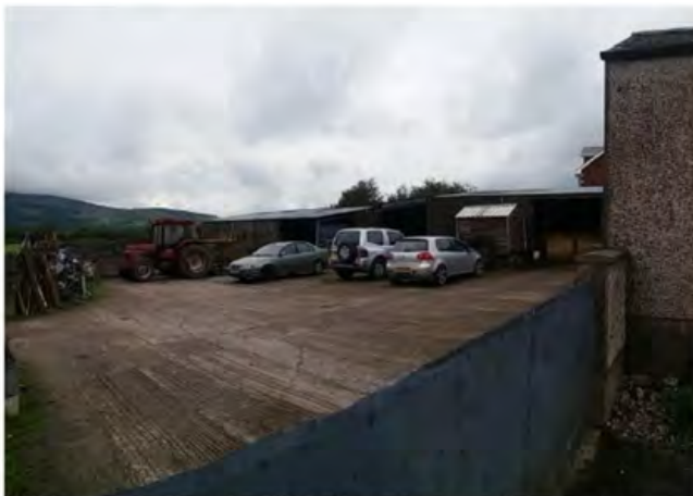
Existing buildings at No.73 Newtown Rd
