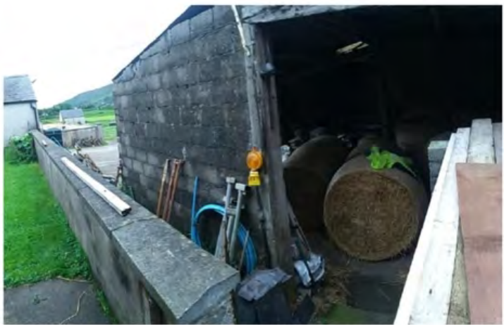
Existing buildings at No.73 Newtown Rd
