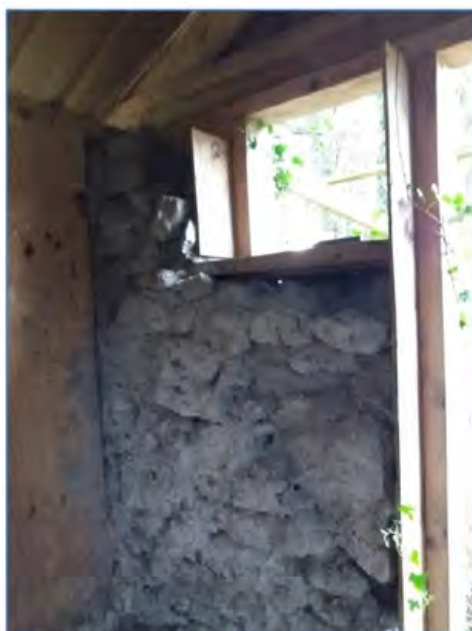
Internal wall, window and door of rear gable wall
