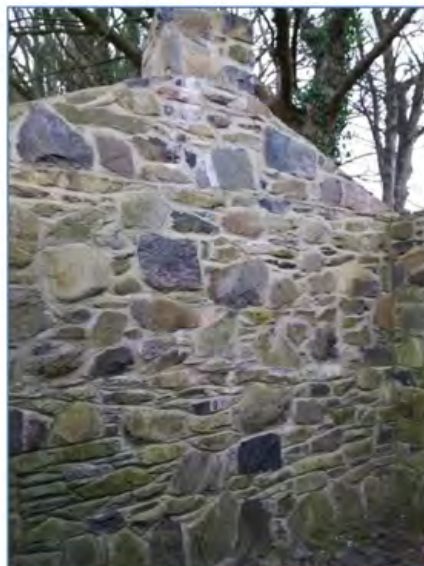
Internal wall of smaller portion of building, no fireplace corresponds with the chimney
