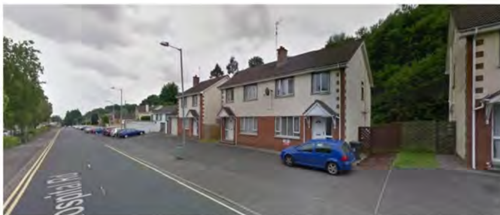
Hospital Road, Newry. Note the gradient of the excavated embankment to the immediate rear of the properties.
