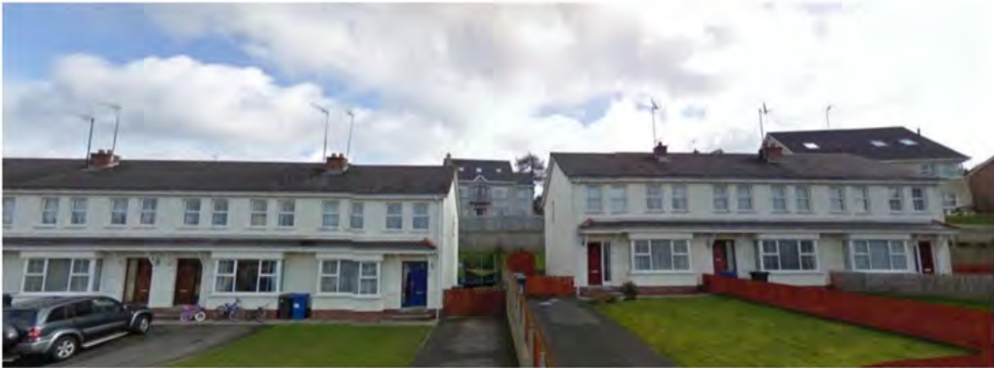
Retaining structures at Carrickdesland, Warrenpoint
