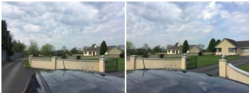
Access to Nos 61 and 63
