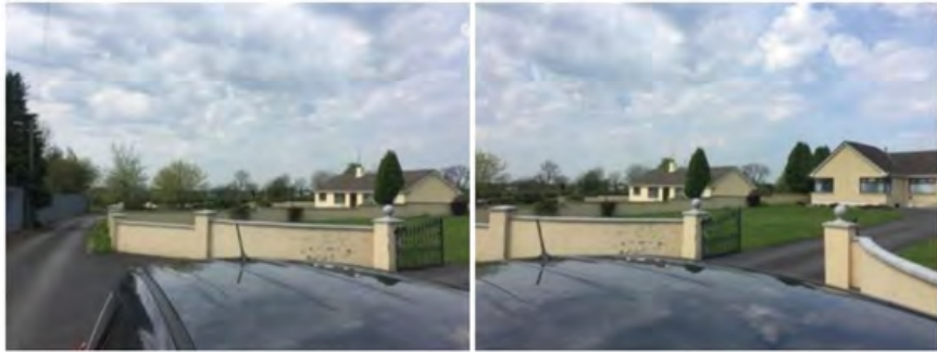
Access to Nos 61 and 63
