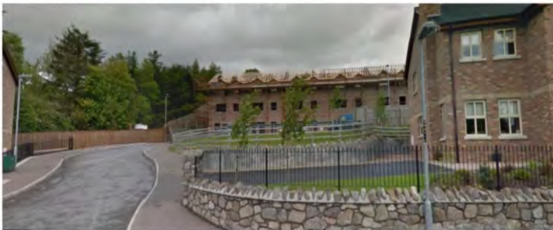
New development at Chapel Road / Commons Way, Newry. Note the extent of the retaining wall to the left of the upper terrace. This retaining structure wraps around the immediate rear of the dwellings in question.
