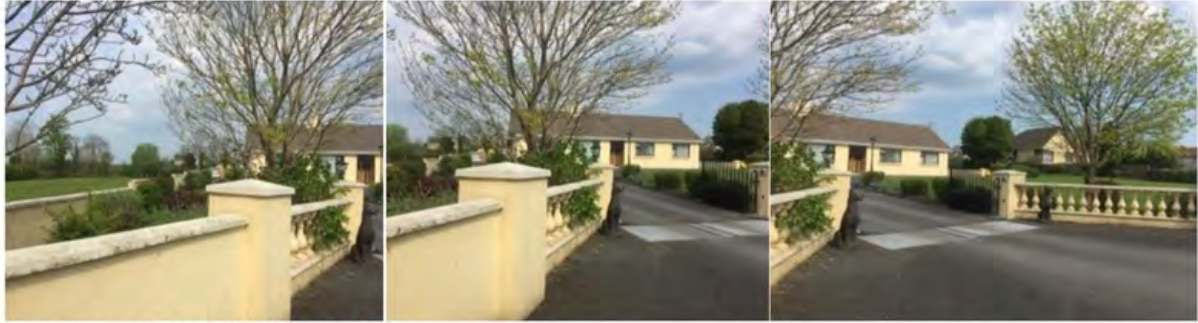
Entrance of No 63 (Site to SW)
