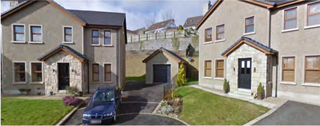
Retaining structures at Greenacorraig, Burren, Warrenpoint.
