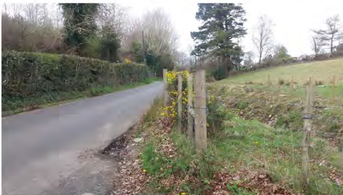
Northern visibility splay blocked by fencing and whin bushes
