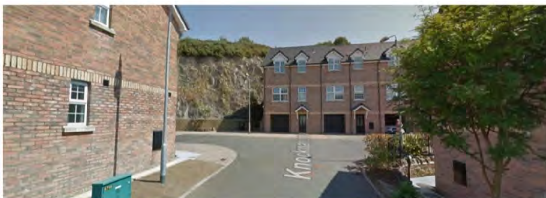
Modern development at O'Neill Avenue, Newry. The extent of the site excavation is apparent, to the left and right of the terraces. The rock face extends along the rear of the dwellings.
