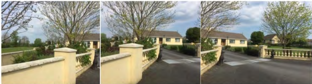
Entrance of No 63 (Site to SW)
