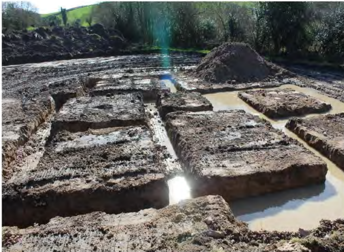
Image 1 - Photographic evidence confirming the demolition of the former dwellings, stripping of topsoil, and the excavation of foundation trenches.
