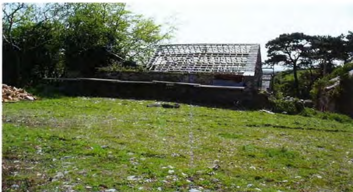
Photograph of rear outbuilding taken by planning officer 2015/16 showing exposed rafters
