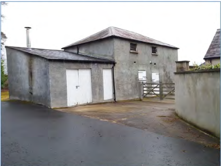
Outbuildings proposed for demolition
