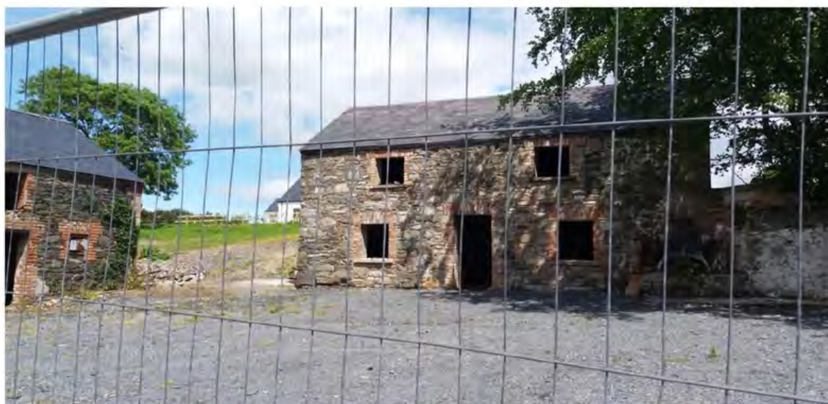
Current form of rear outbuilding. Photograph taken by planning officer June 2017 showing new opening on front elevation and introduction of red brick.
