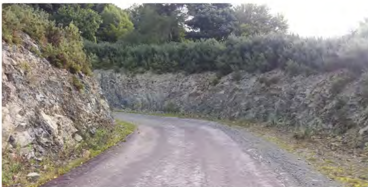
Existing access lane
