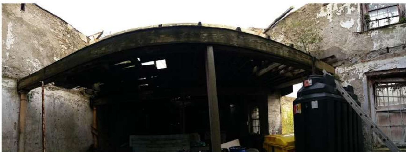
Existing storage building to be used for distillery area
