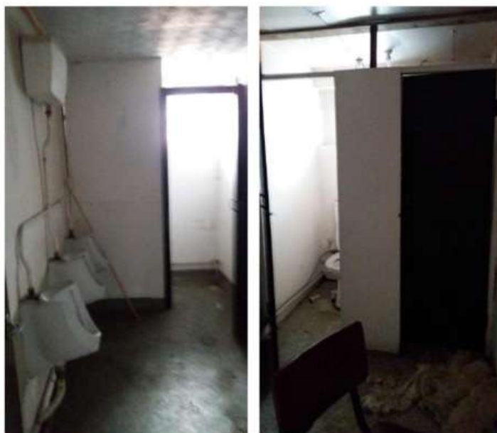
Existing toilet area at 1 st floor level to be removed and area used as part of theatre/ function room
