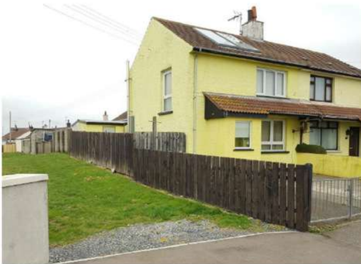
Front elevation of No. 1 Seaview
