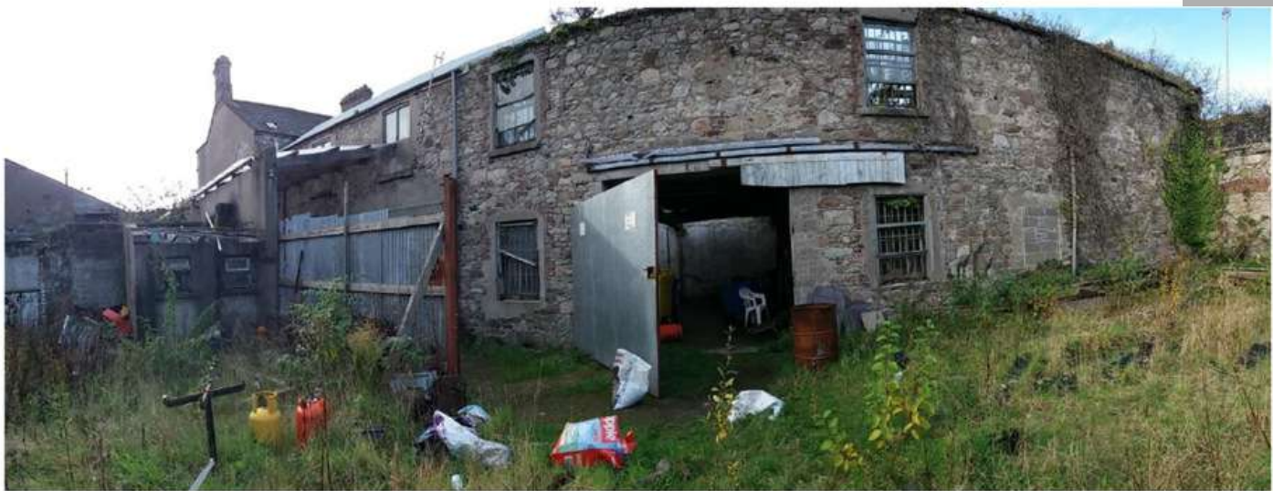
Existing storage building to be used for distillery area
