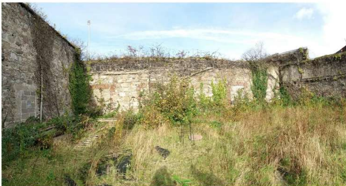
Existing rear yard
