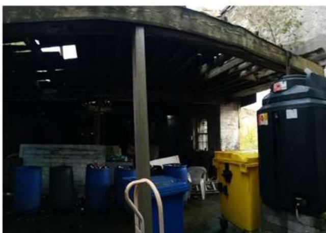
Existing storage building to be used for distillery area
