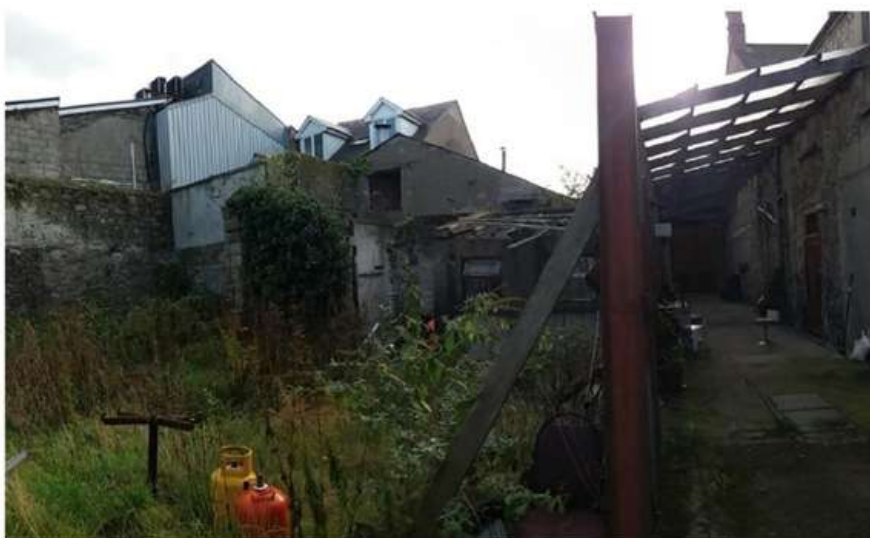
Existing rear yard
