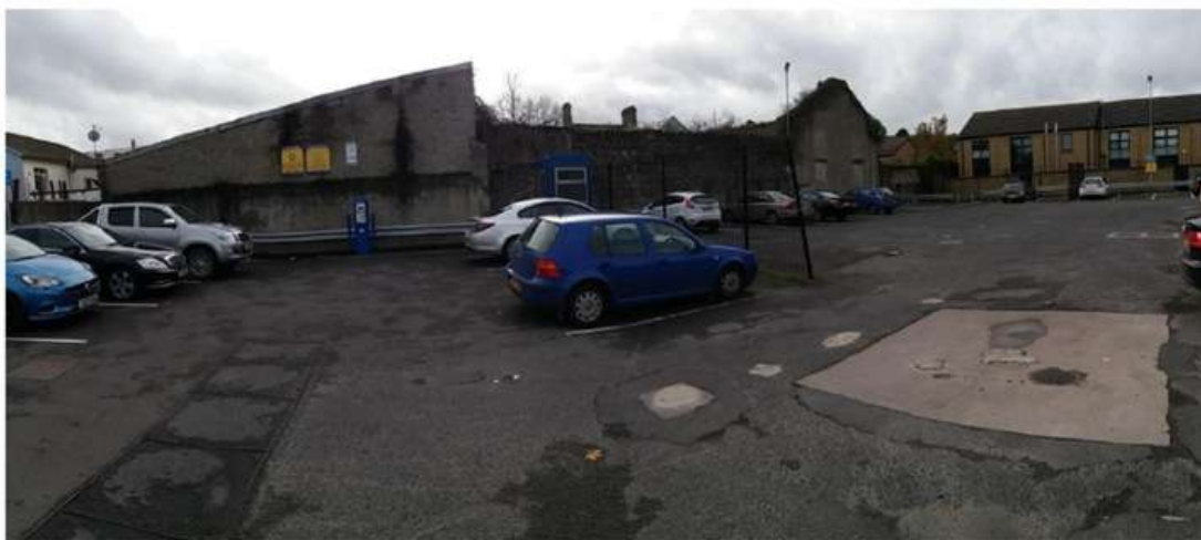
Existing car park to rear of property, rear elevation of existing buildings
