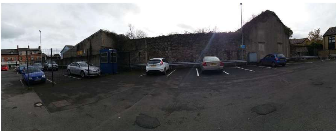
Existing car park to rear of property, rear elevation of existing buildings
