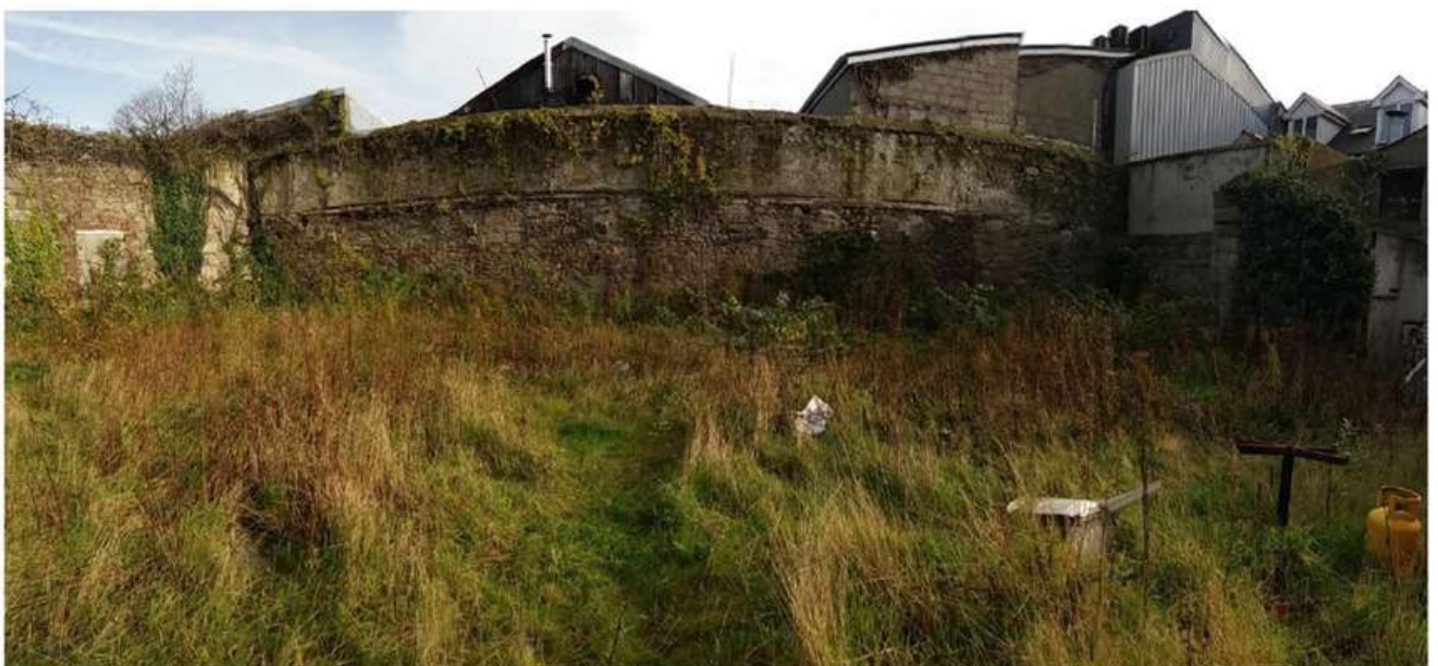
Existing rear yard
