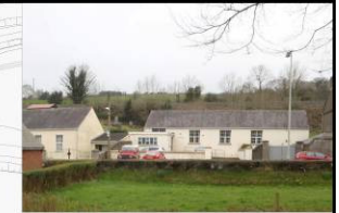
Extension to the Village Hall to facilitate a greater variety of uses.
