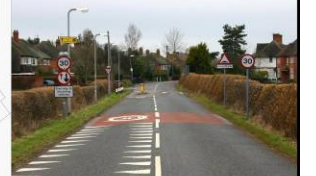
New entrance signs, advisory 40mph speed limit and crossing point to facilitate pedestrian access between the village and the canal.
