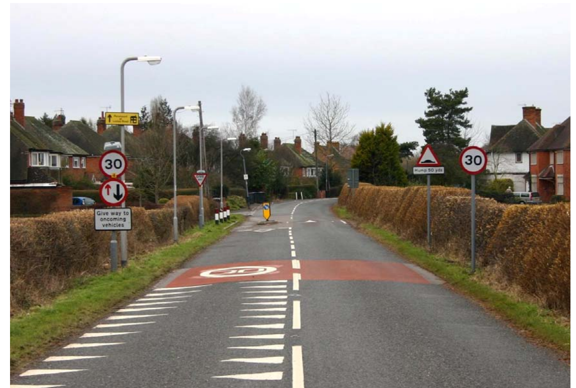
Road markings, signage and speed humps.
