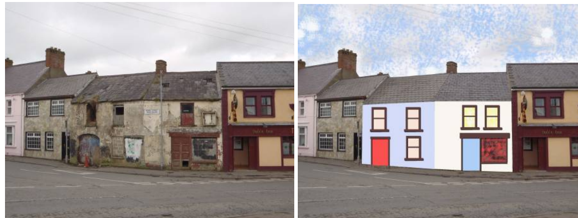
Figure 3.11: Sprucing up vacant and derelict buildings can be as simple as a paint scheme in the short term.
