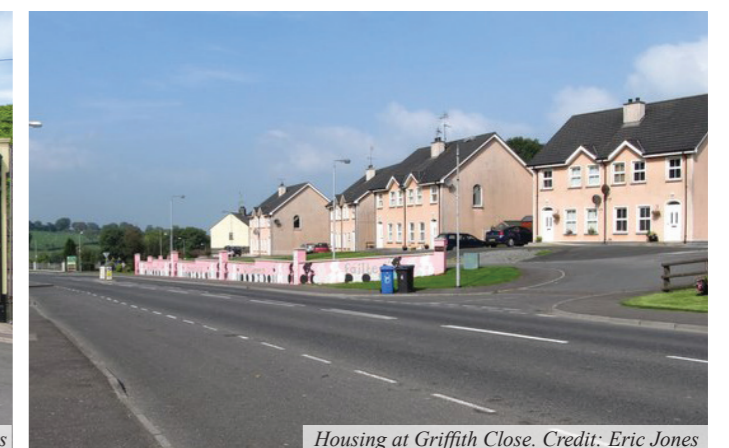
Housing at Griffith Close. Credit: Eric Jones
