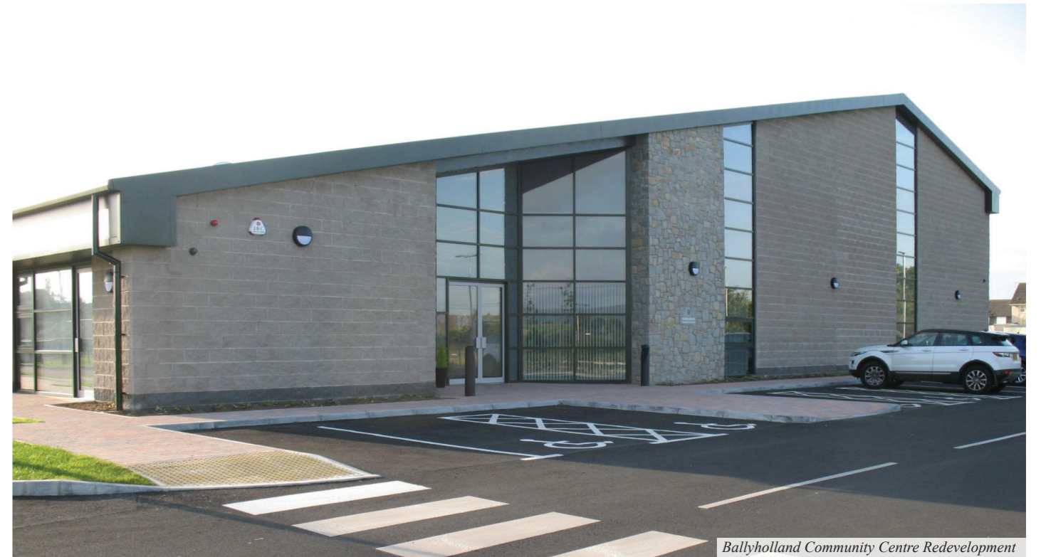
Ballyholland Community Centre Redevelopment
