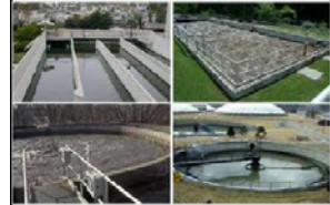
Improved sewerage system installed to cope with village needs.
