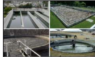
Improved sewerage system
