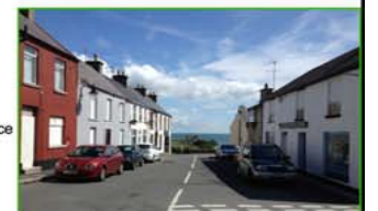
Main Street vacant properties already painted.
