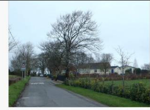
Provision of street lighting along Cortamlet Road in front of the Primary School and Church.
