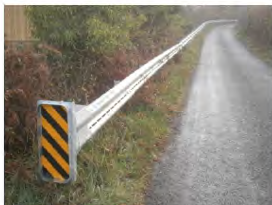
The start of the new VRS on Flagstaff Road
