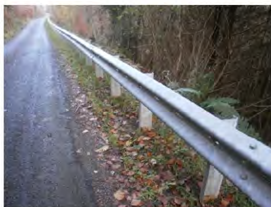
A section along the new length installed
