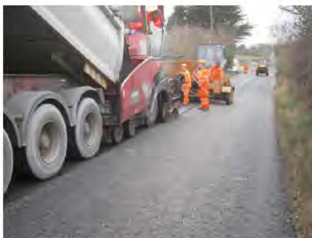
Asphalt resurfacing being carried out within the Division
