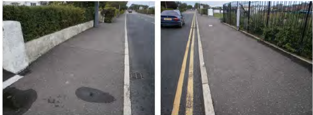
The newly widened footways along both sides of Shimna Road at the end of resurfacing works
