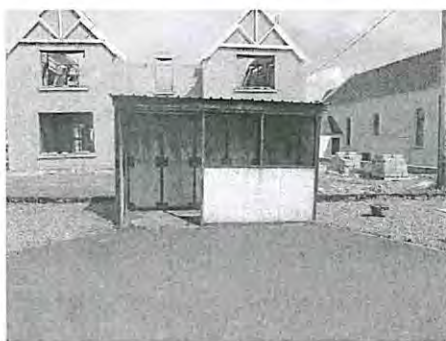
Existing bus shelter fronting dwelling
