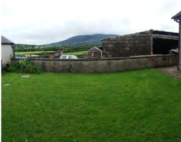
Existing buildings at No.73 Newtown Rd
