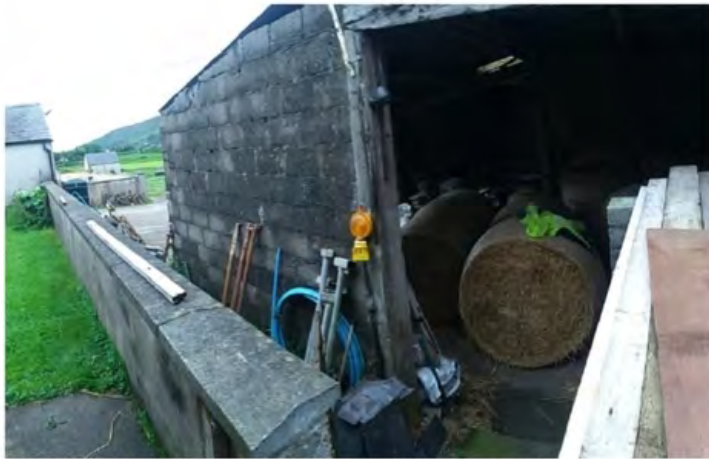
Existing buildings at No.73 Newtown Rd
