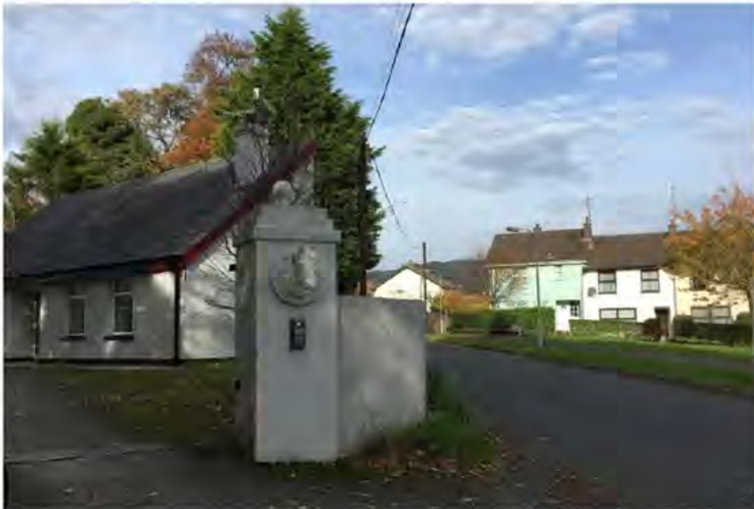
Figure 5: Substandard View North from Existing Access
