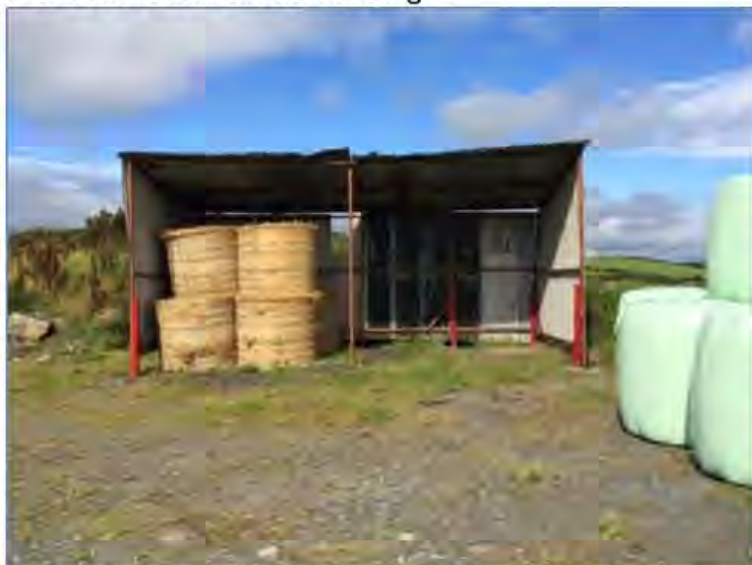
Front elevation of the building
