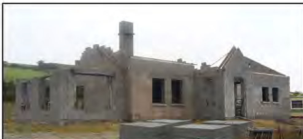
Figure 1 - Dwelling Under Construction
