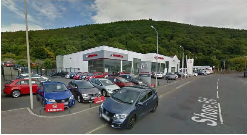
Figure 6: Existing Car Showroom
