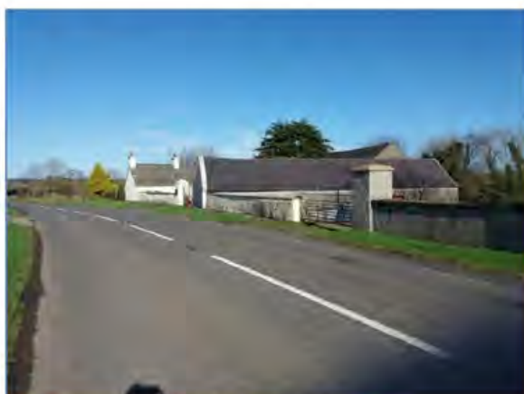
View of the site from the South
