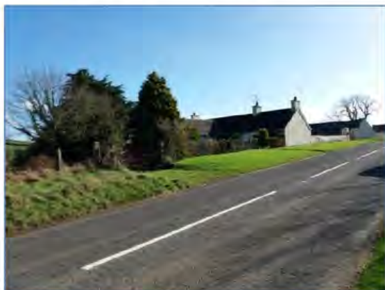
View of the site from the North
