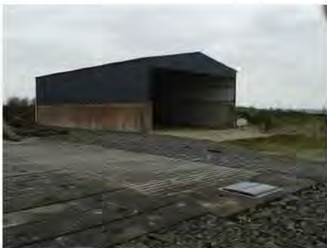
Fig 3: Slurry tank and agricultural building located south-west of the application site
