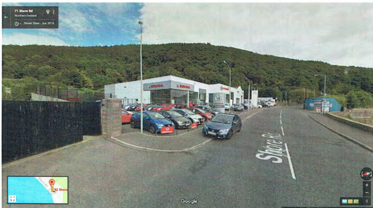
Figure 3: Existing Car Showroom on Site
