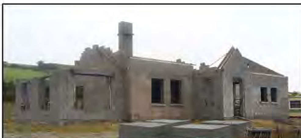
Figure 1 - Dwelling Under Construction
