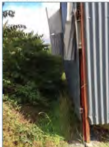
Rear of the structure
