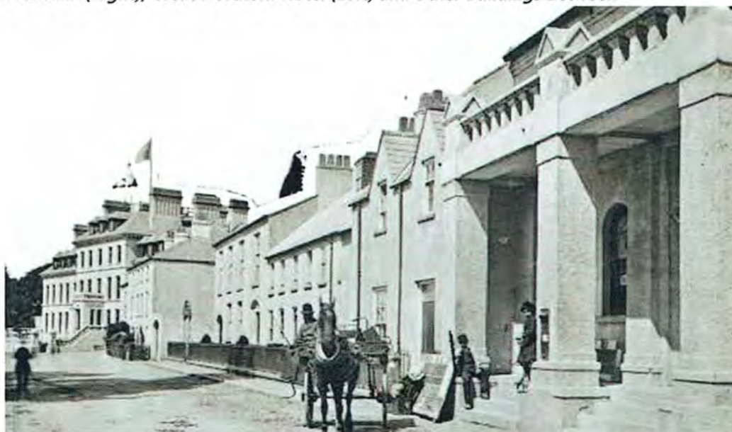
Figure 1: Ice Rink (Right), Great Northern Hotel (Left) and Other Buildings Between
