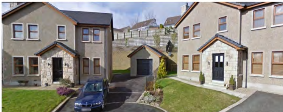
Retaining structures at Greenacorraig, Burren, Warrenpoint.
