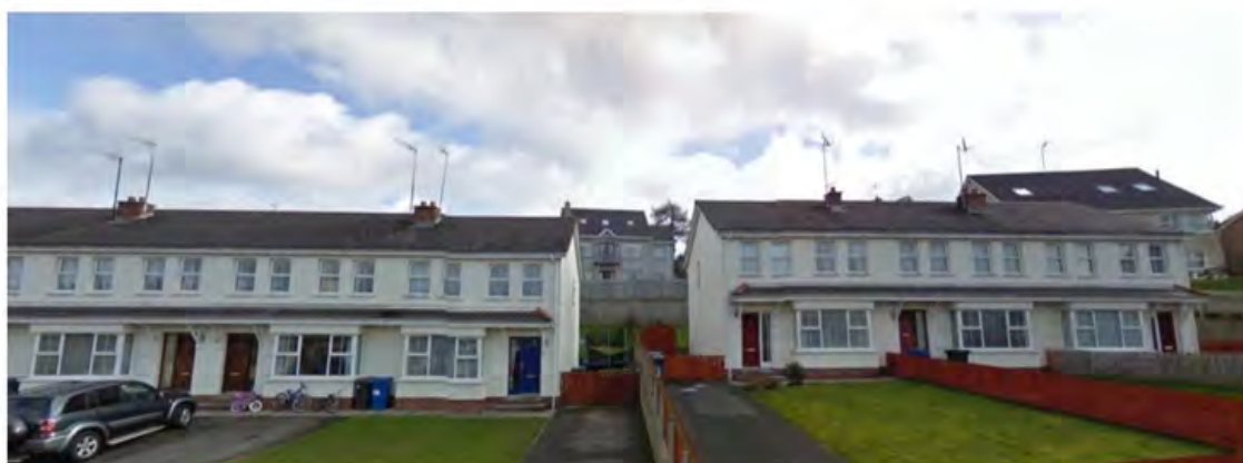
Retaining structures at Carrickdesland, Warrenpoint
