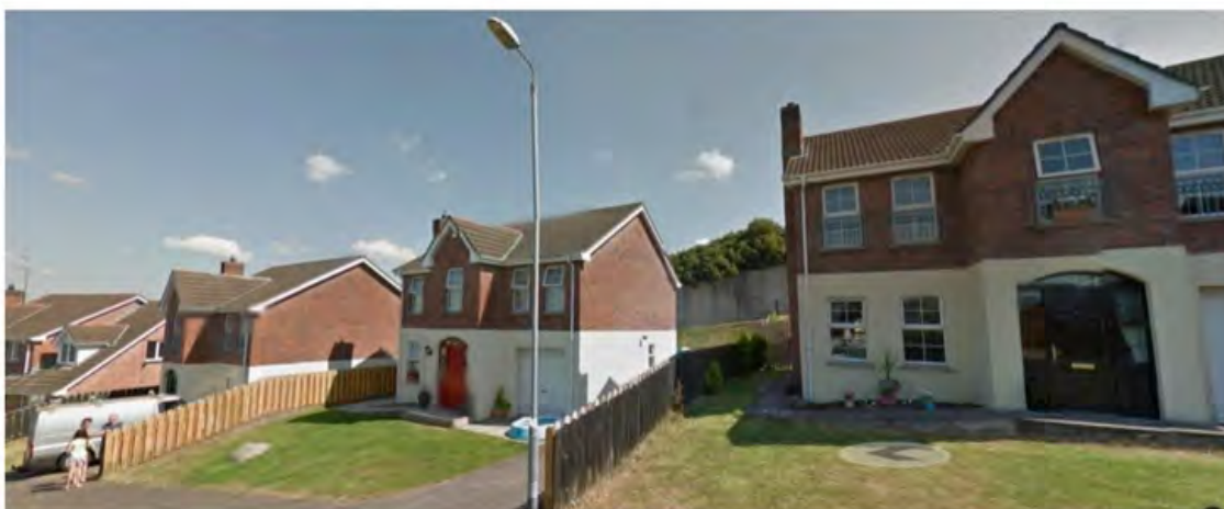
Knockdarragh, Newry. Note the retaining structures to the rear of the dwellings in question. Note also the retaining structures between individual rows of dwellings.
