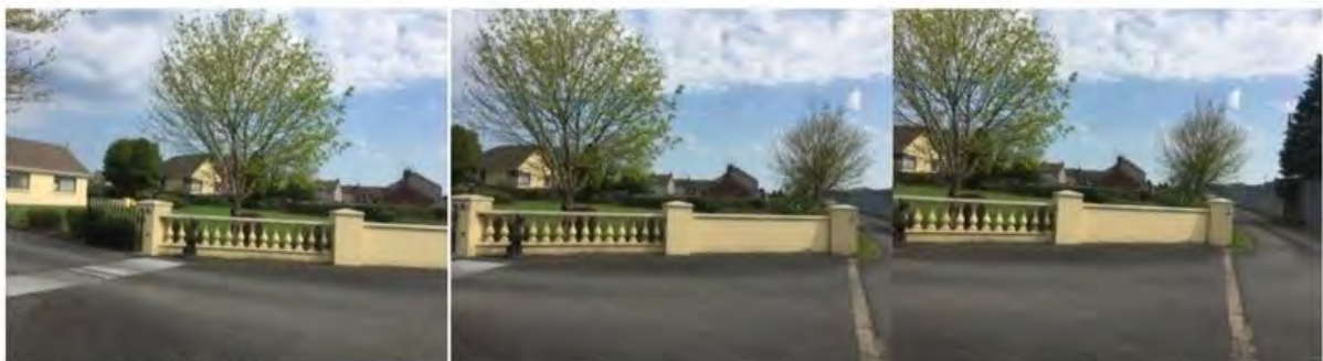
Entrance of No 63
