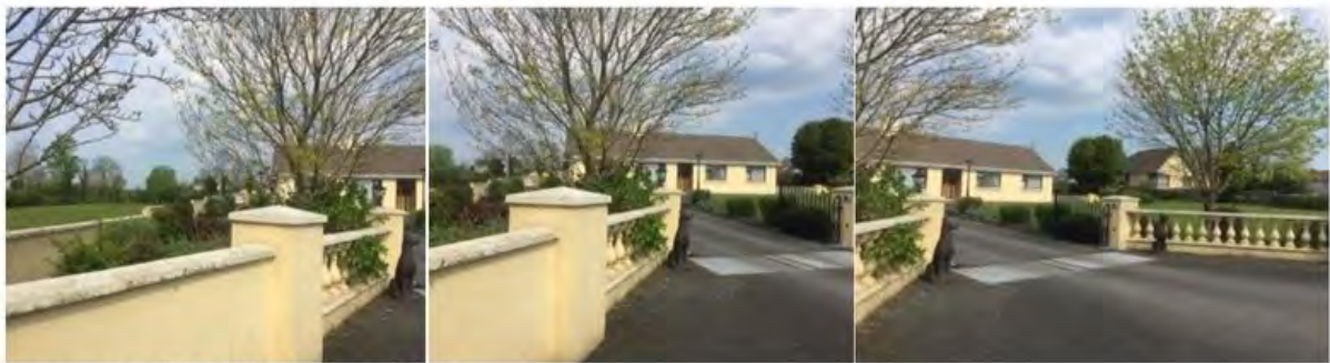
Entrance of No 63 (Site to SW)
