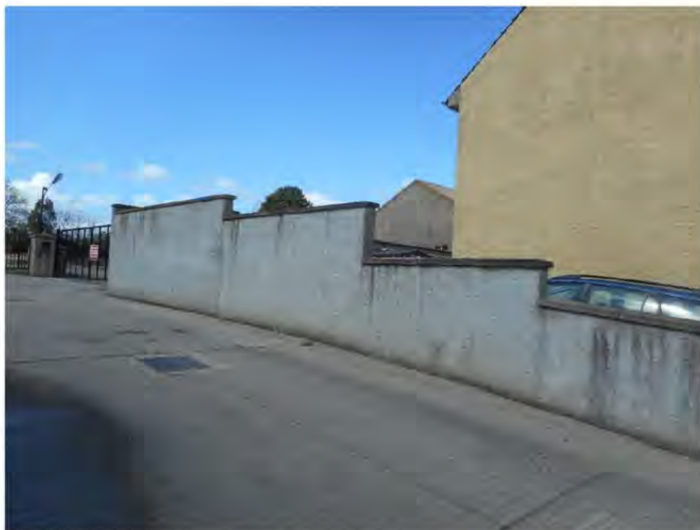
Photo 6 – Wall and Blank gable of No.4 Austin Terrace
