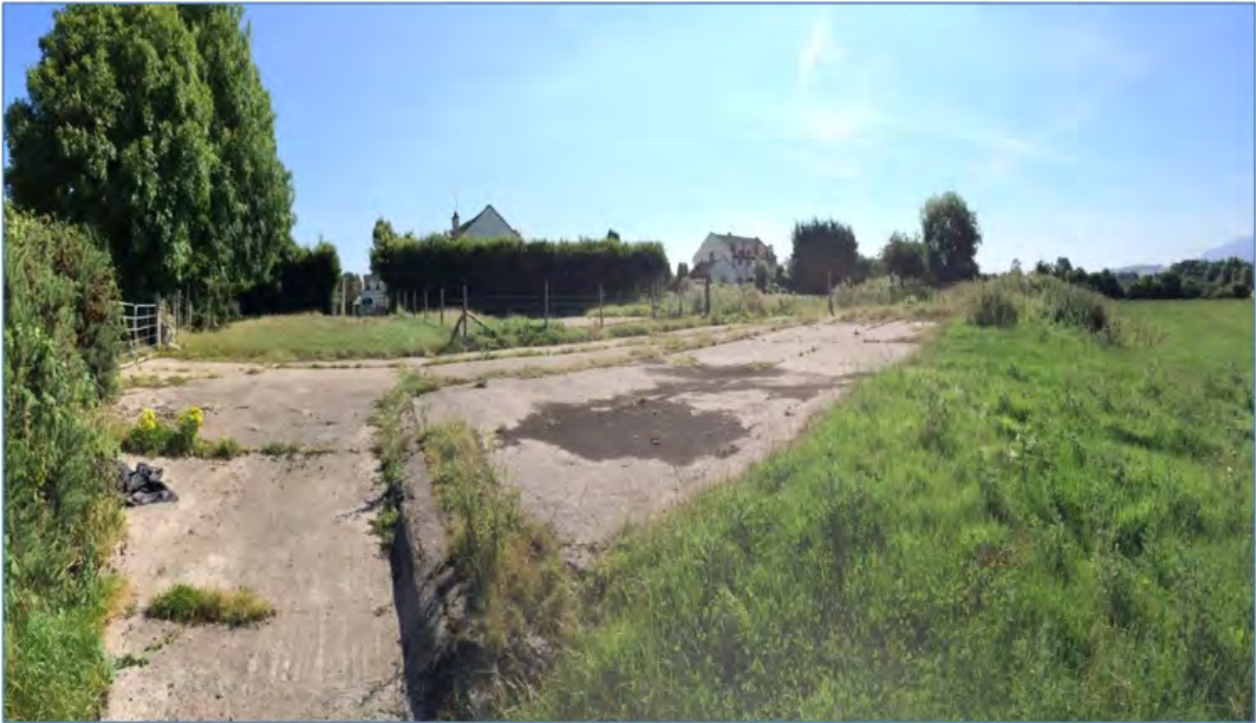
View of the site from the NE corner (internal view)
