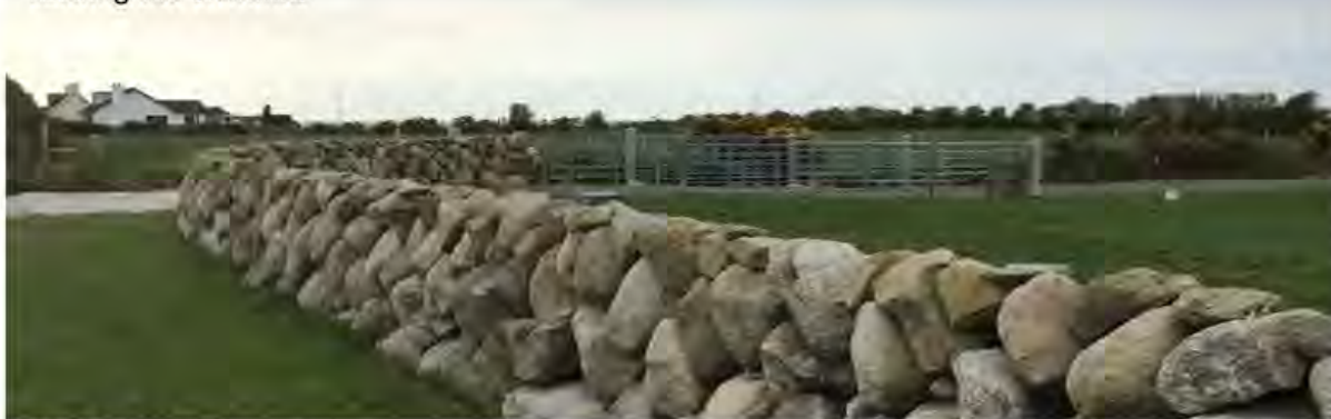
Existing site entrance
