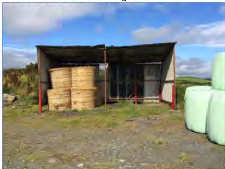
Front elevation of the building
