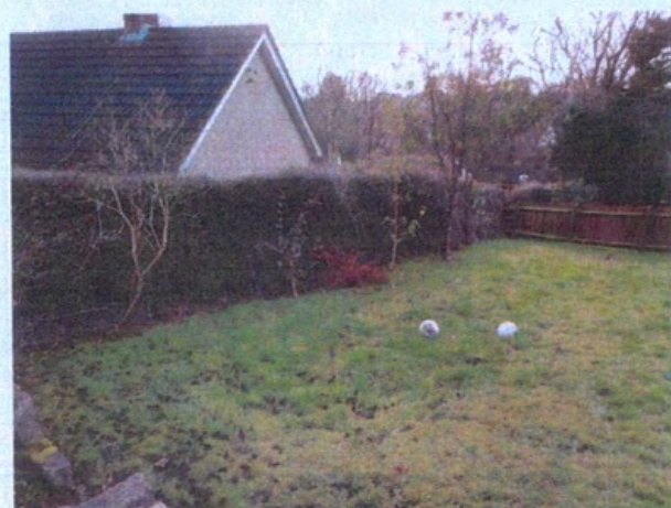
Photo 6 – No.10's Blank Gable
