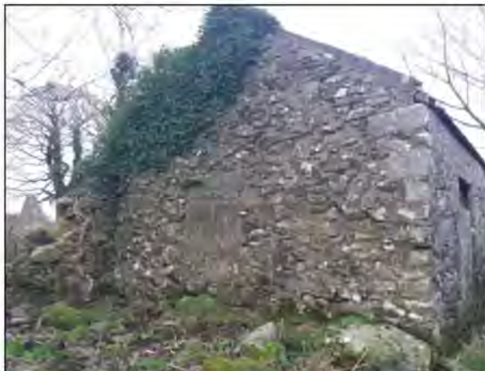
Figure 4 - Original Gable End
