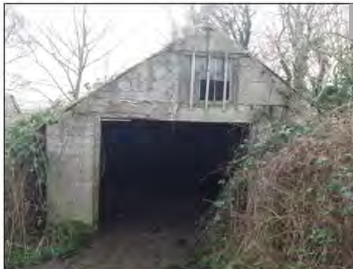
Figure 3 - Block Built Gable End
