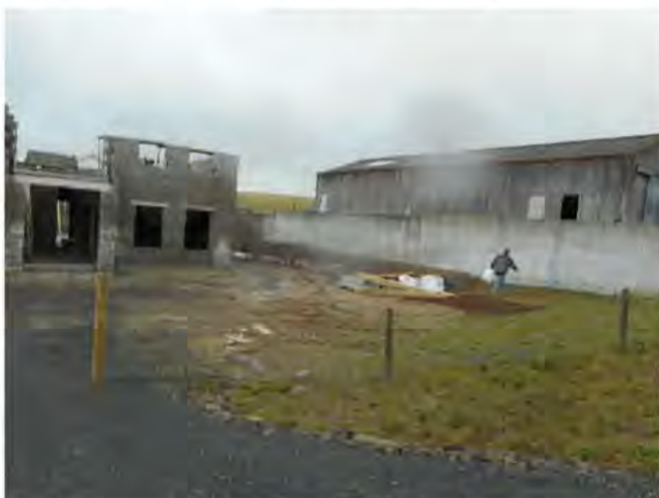
Photo 12 – Byre and new dwelling under construction
