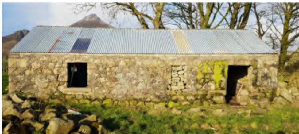
Photo No 1. Front elevation showing 2 windows and a door opening to the right side.
