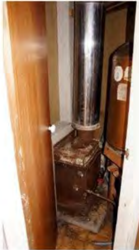
Central heating boiler
