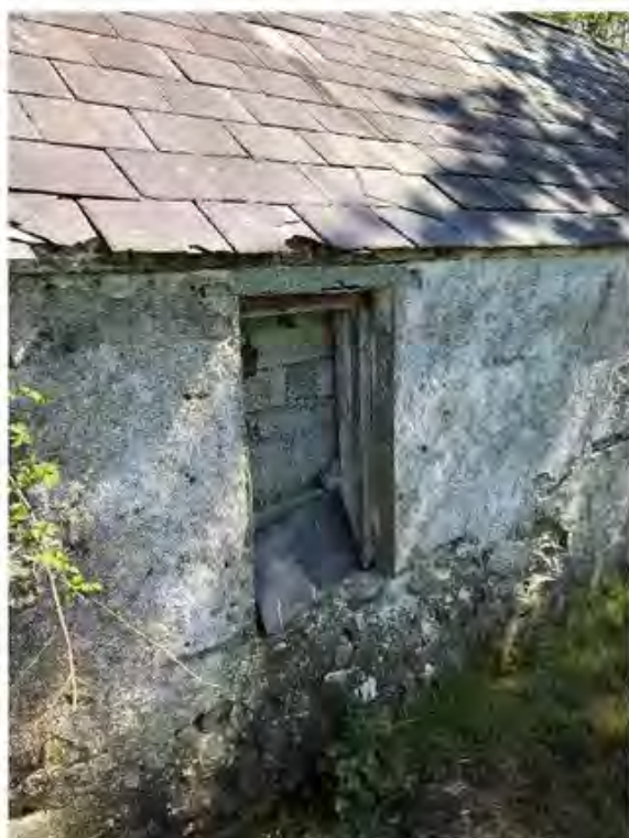
Existing building with domestic features and finishes
