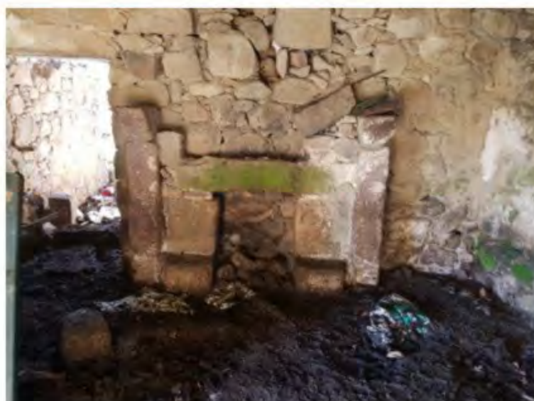
Photo No 2. Internal photo showing the original fireplace with the connecting door between 2 internal rooms.
