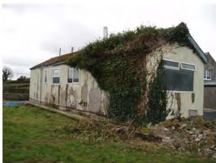
Side elevation of Structure
