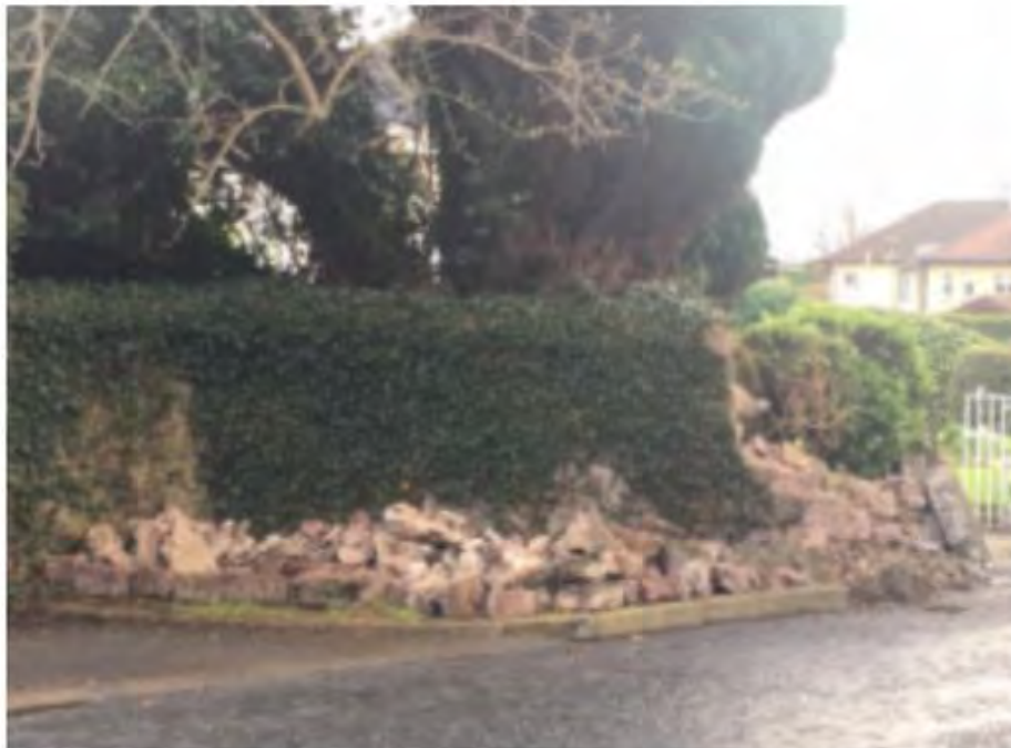
A very badly damaged stone wall at Well Road
