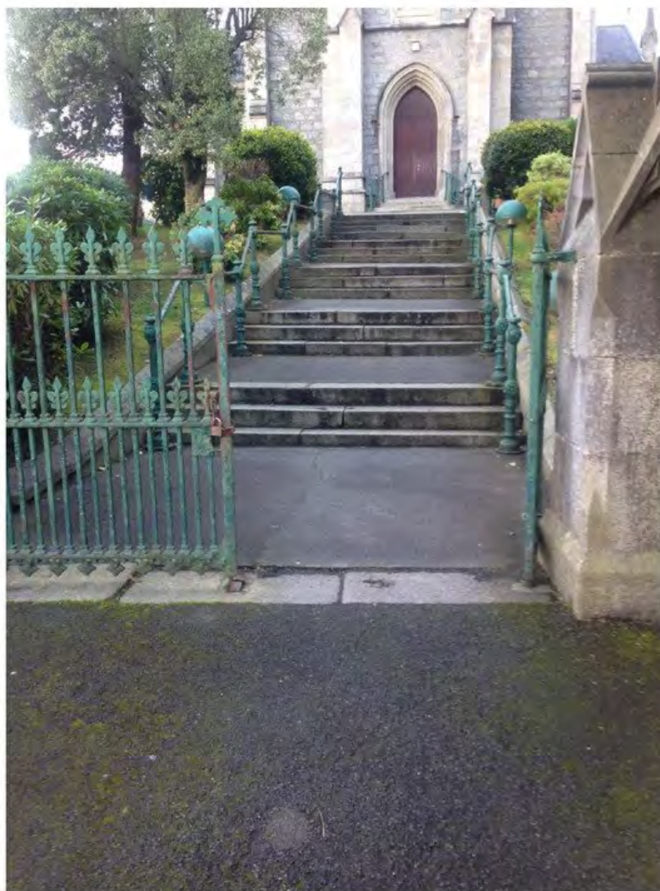
Steps to Church with associated railings.
