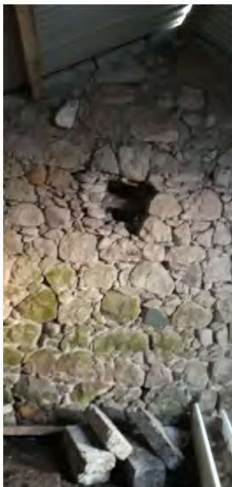
Photo No 4. Internal photo taken 17/12/2018 showing the wall behind the channel. The wall has no sign of vertical joints which would be visible if a window opening was built up as the officer suggests.
