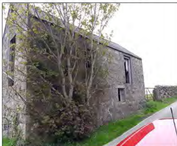
Building to be converted
