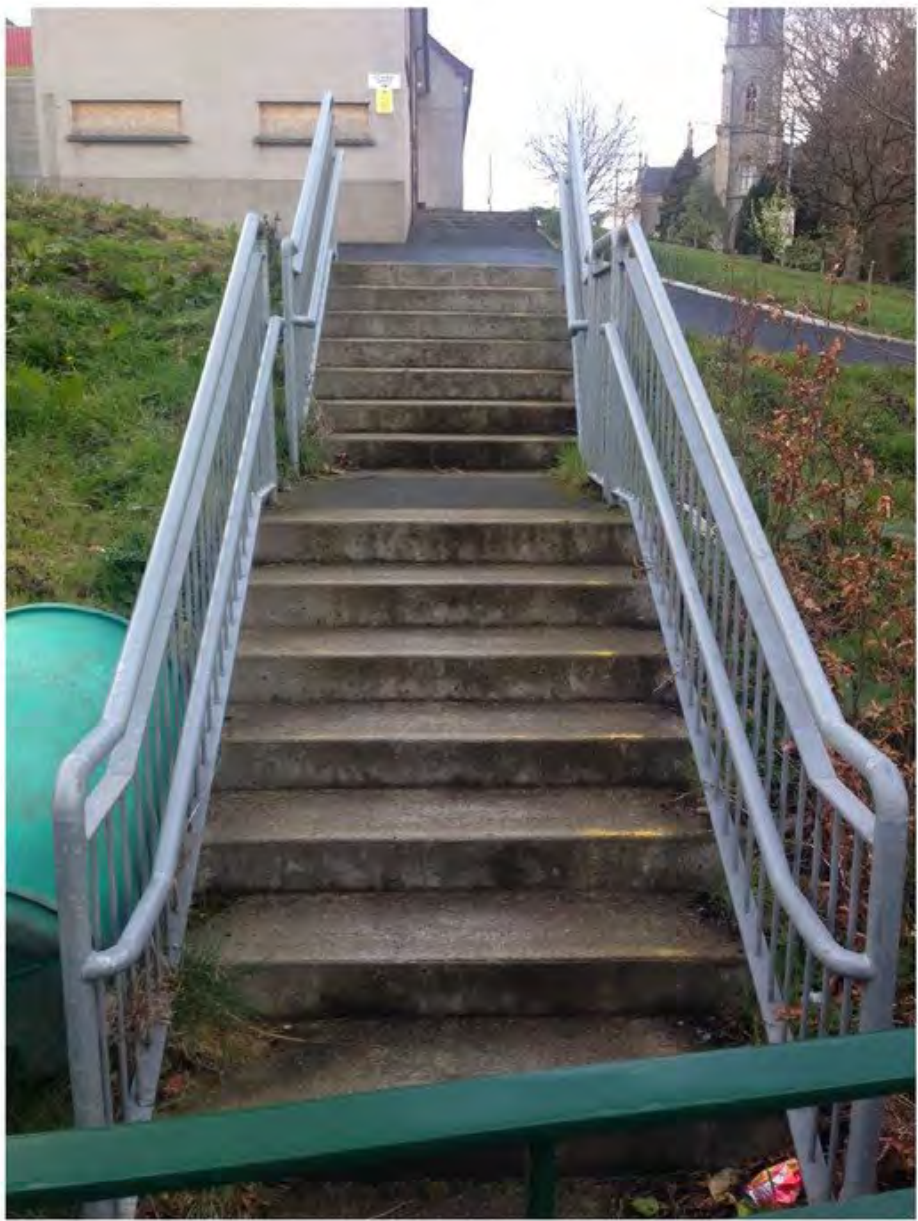
More steps and railings opposite our site
