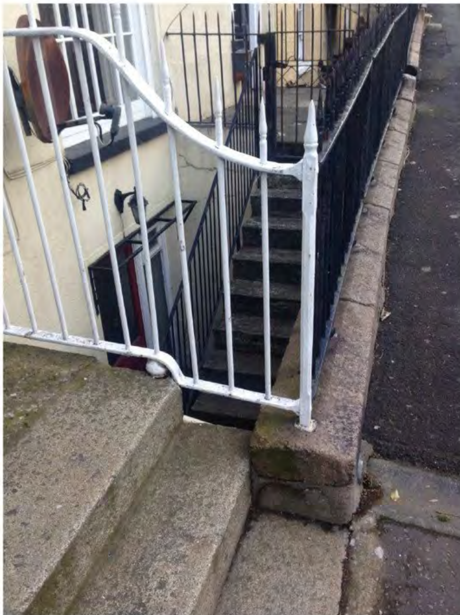
Steps and railings at building on entrance to village from Warrenpoint side
