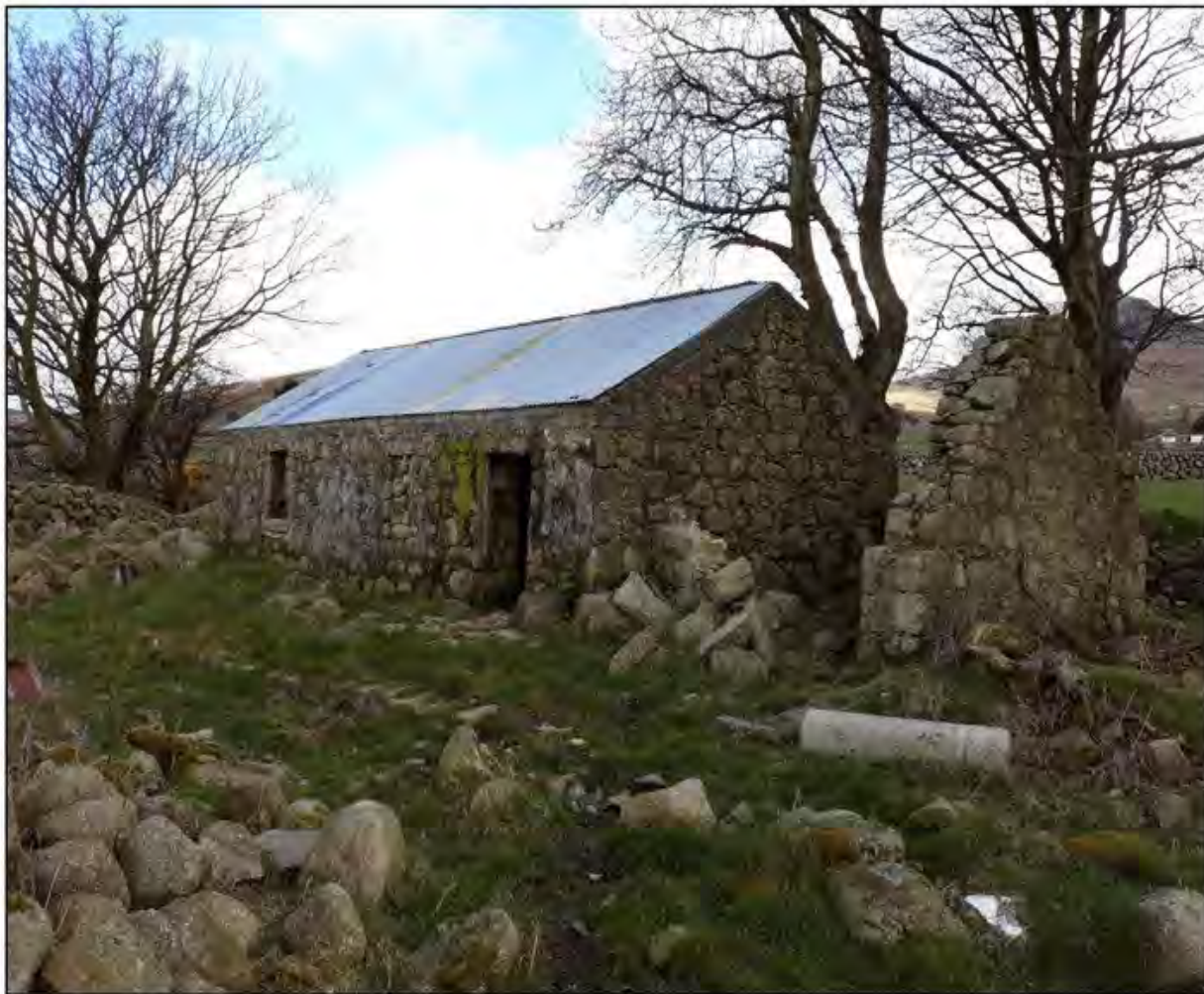
Building to be replaced
