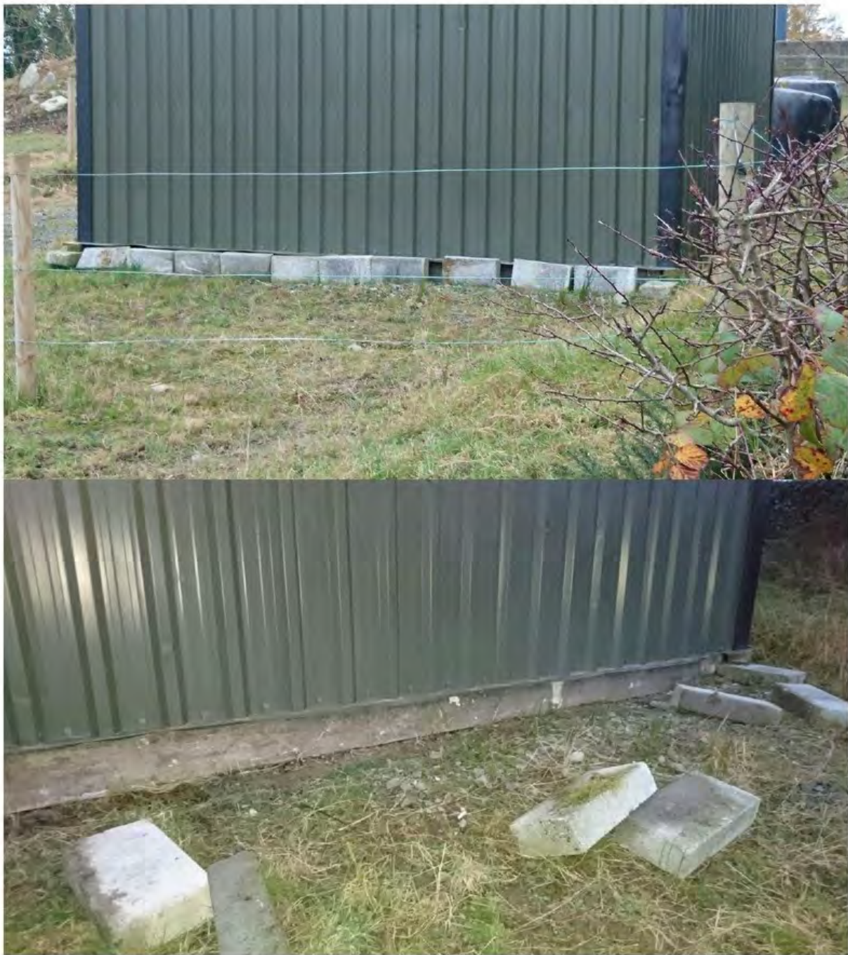
App 6 – Various Photographs – Blocks retaining base shuttering timbers – Internal and external shots. Sheep feeding, neighbouring workshop, yard and shed.
