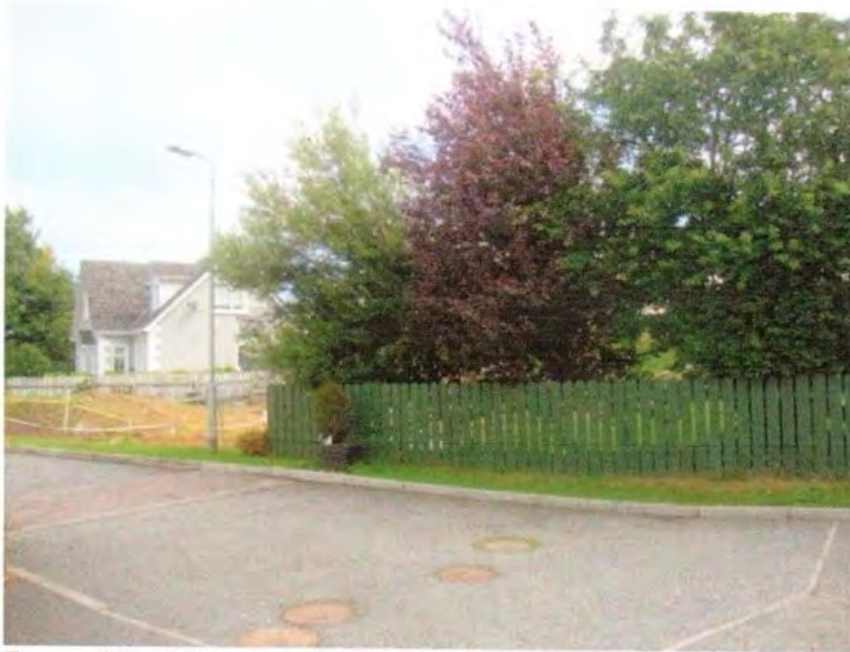
Front of No. 8 Mayvale looking E (Plots to rear of 1 and 2 Whinnbloom visible)
