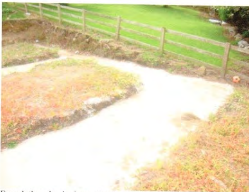
Foundations in site immediately adjacent and north (note level differences)
